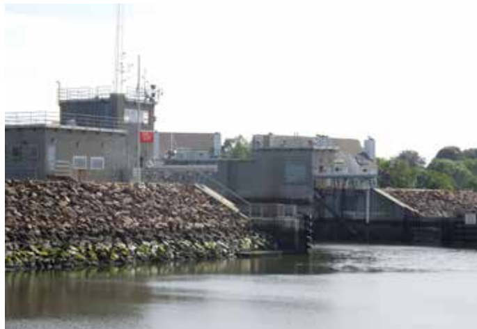
Stamford Hurricane Barrier in Connecticut.
