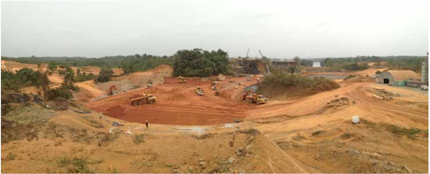
Work at the Mount Coffee Hydropower Plant in Liberia is ongoing. The project will supply much needed power and clean water to local residents.
