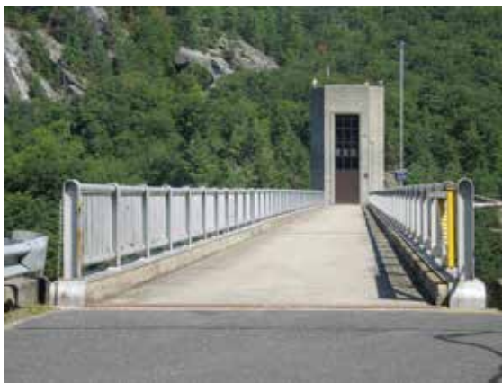
Ball Mountain Dam in Vermont.
