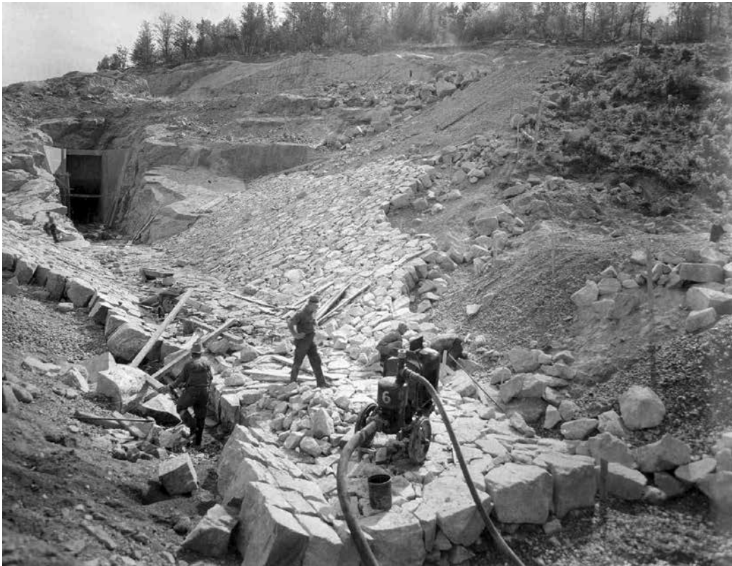
Construction workers labor to build the $2.8 million Surry Mountain Dam project in Surry, New Hampshire in this circa 1942 photo.
