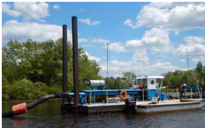
Dredging Milford Pond in Milford, Massachusetts.
