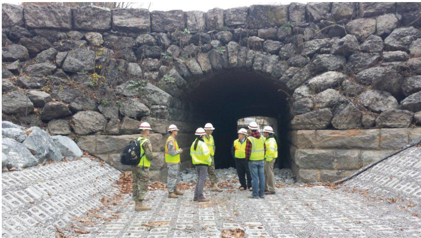
Brig. Gen. Graham (center) gets a tour of the Muddy River Project in Boston, Massachusetts.
