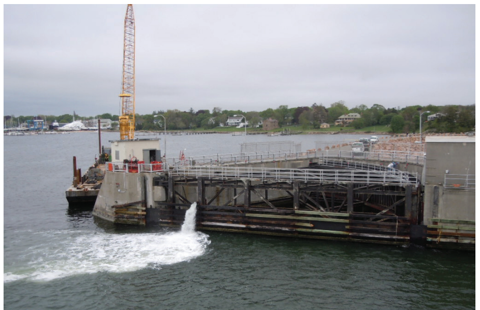
New Bedford Hurricane Barrier.
