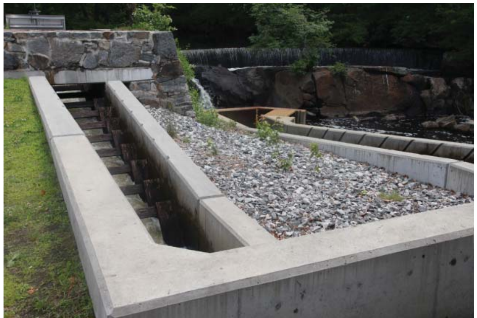
One of the fish ladders that was constructed along the Ten Mile River.
