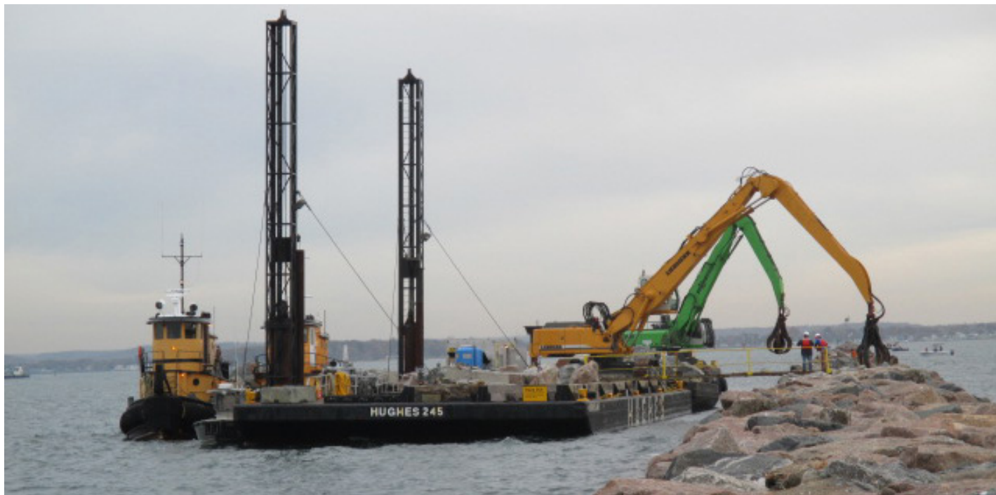
District contractor Mohawk Northeast performs breakwater repairs at New Haven Harbor.
