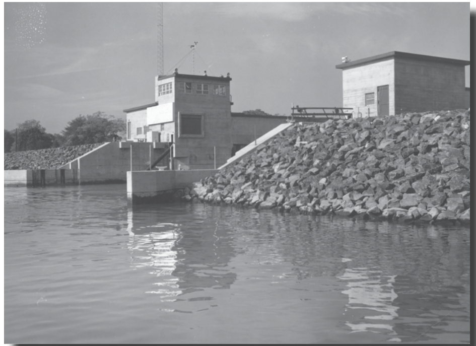
Aerial view of Stamford Hurricane Barrier.
