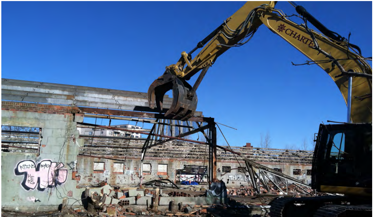
Buildings are demolished as part of the remedial action plan for the Watertown GSA Formerly Used Defense Site.
