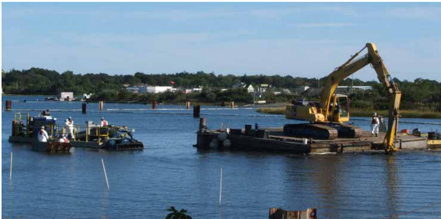
Dredging operations at the New Bedford Harbor Superfund Site.
