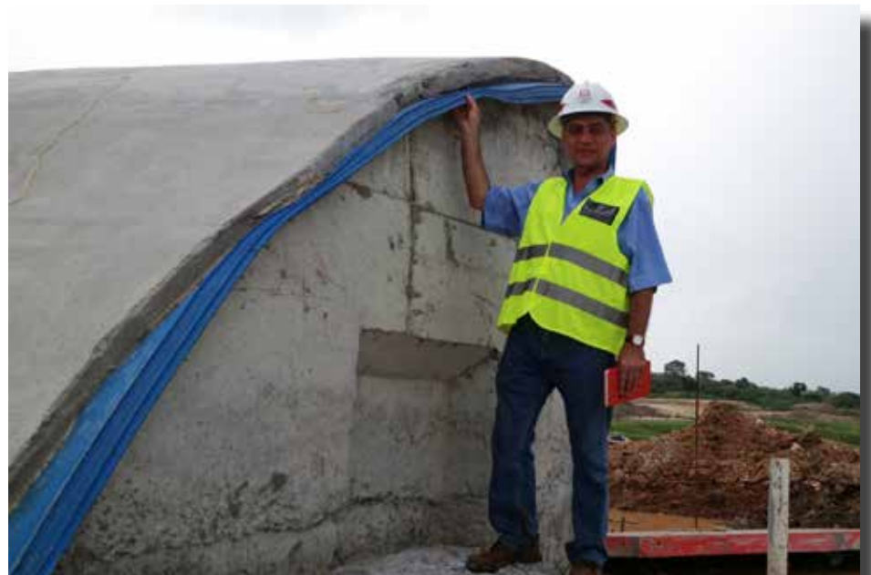
Siamac Vaghar at the Nacala Dam Construction site in Africa.
