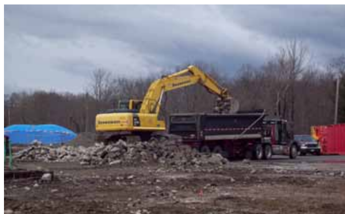
Construction at the Hatheway & Patterson Superfund Site.
