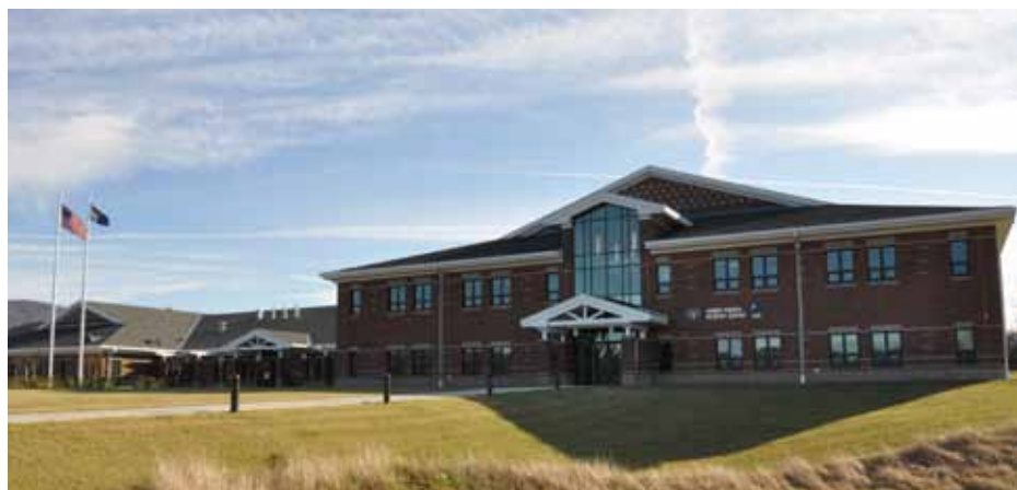
New facility constructed under BRAC in Rutland, Vermont.
