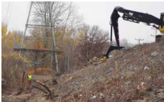
Vegetation removal at Woonsocket Fall Dam in Rhode Island.
