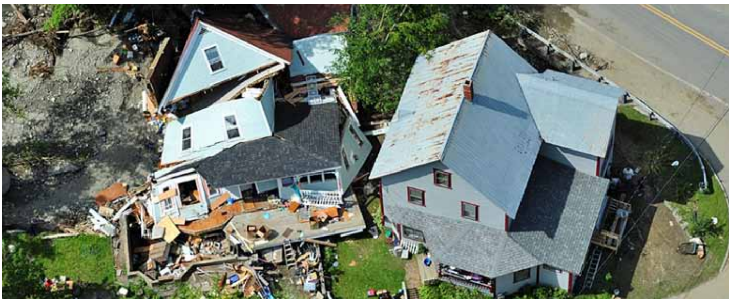
Aerial photo of damage caused by Hurricane Irene in Vermont.
