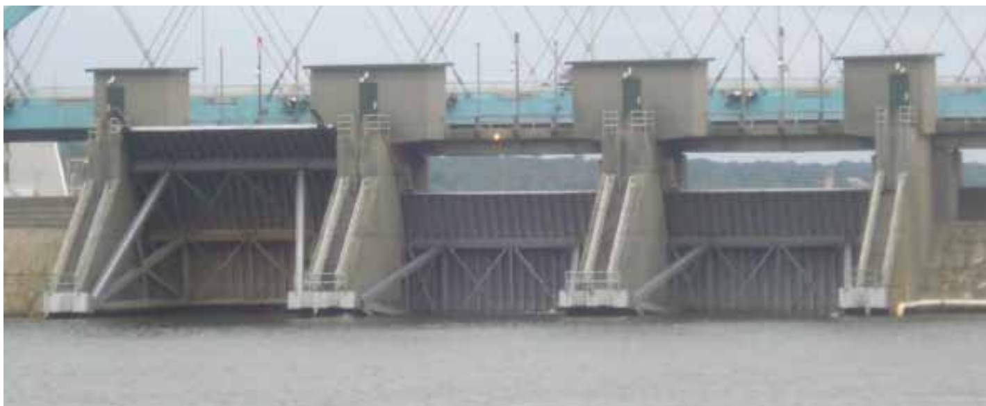
The gates at the Fox Point Hurricane Barrier in Rhode Island closed during Hurricane Irene.
