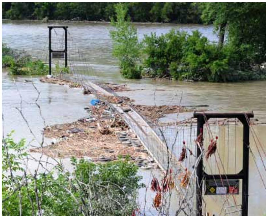
The VAST snowmobile bridge near Waterbury flexes as debris and water rush past.
