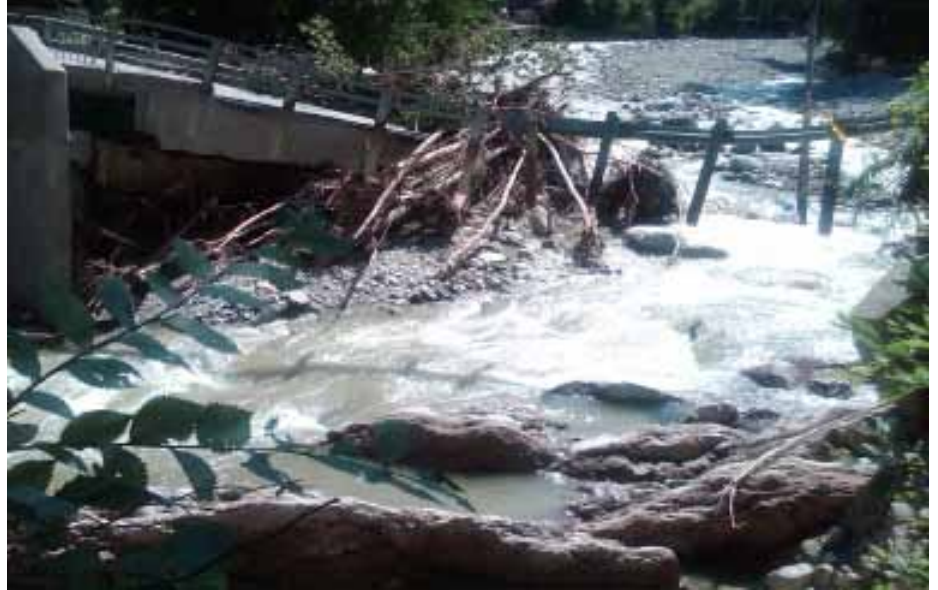
Irene washes out a bridge in Jamaica, Vt., near the District's Ball Mountain Lake Project.
