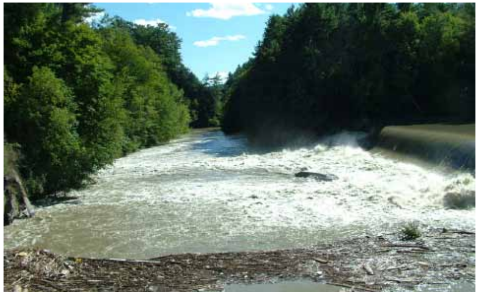
Waters at North Hartland Dam, Vt., after the storm.
