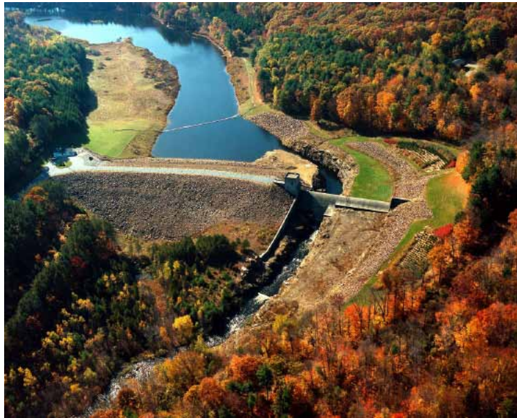
Westville Lake Dam
