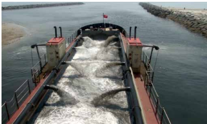
Sediment is pumped into the CURRITUCK's hopper.
