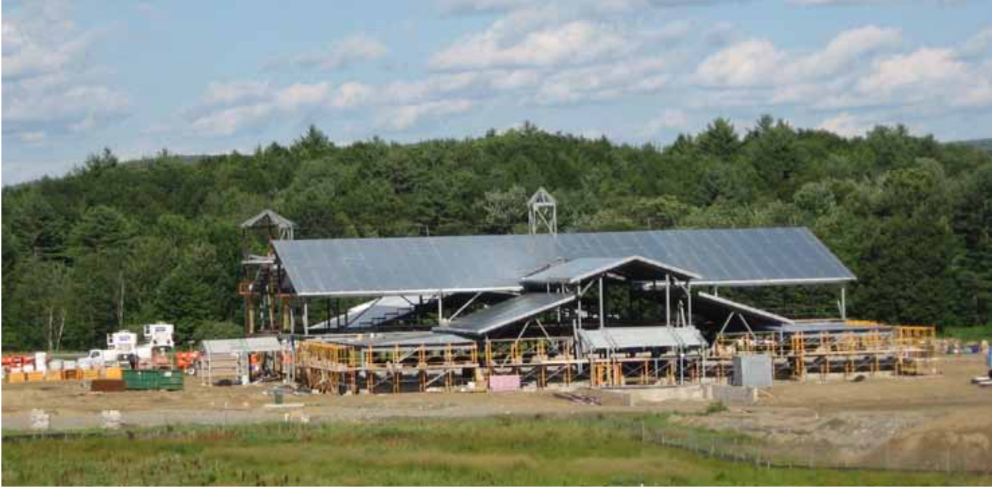
Construction work at the Armed Forces Reserve Center in White River Junction, Vt.
