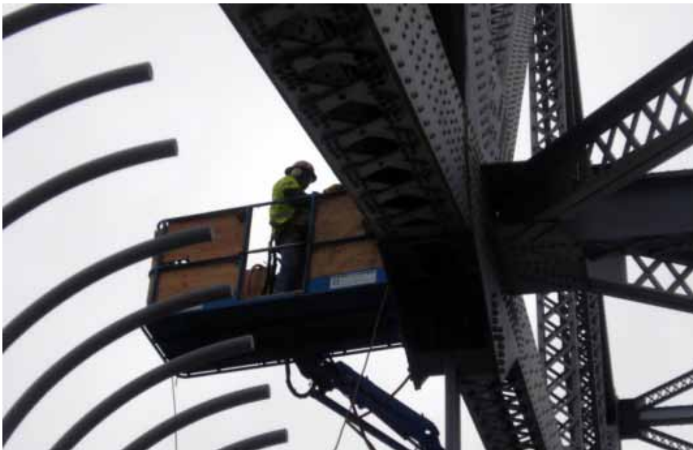
Bourne Bridge construction work.
