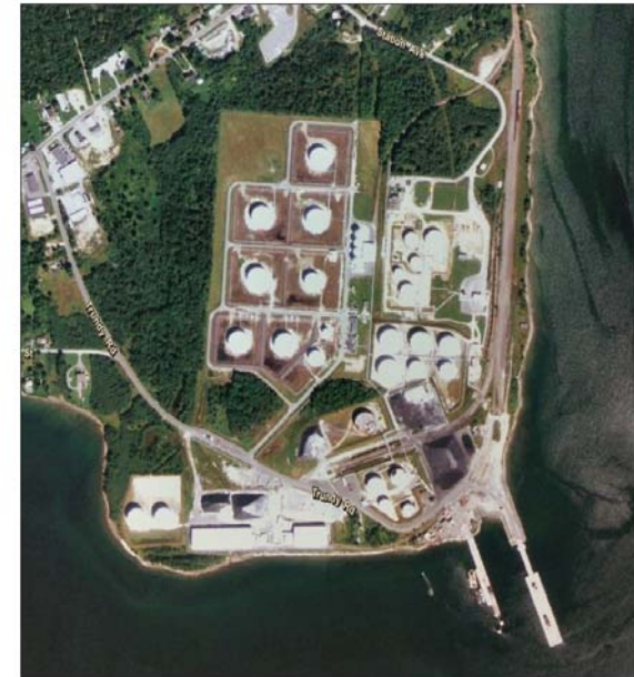
Facilities at Mack Point
