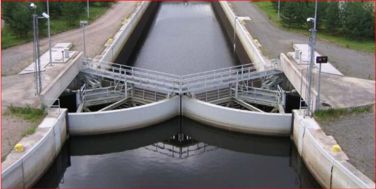
Figure 5-5. Storm surge barrier example (sector gate type)
