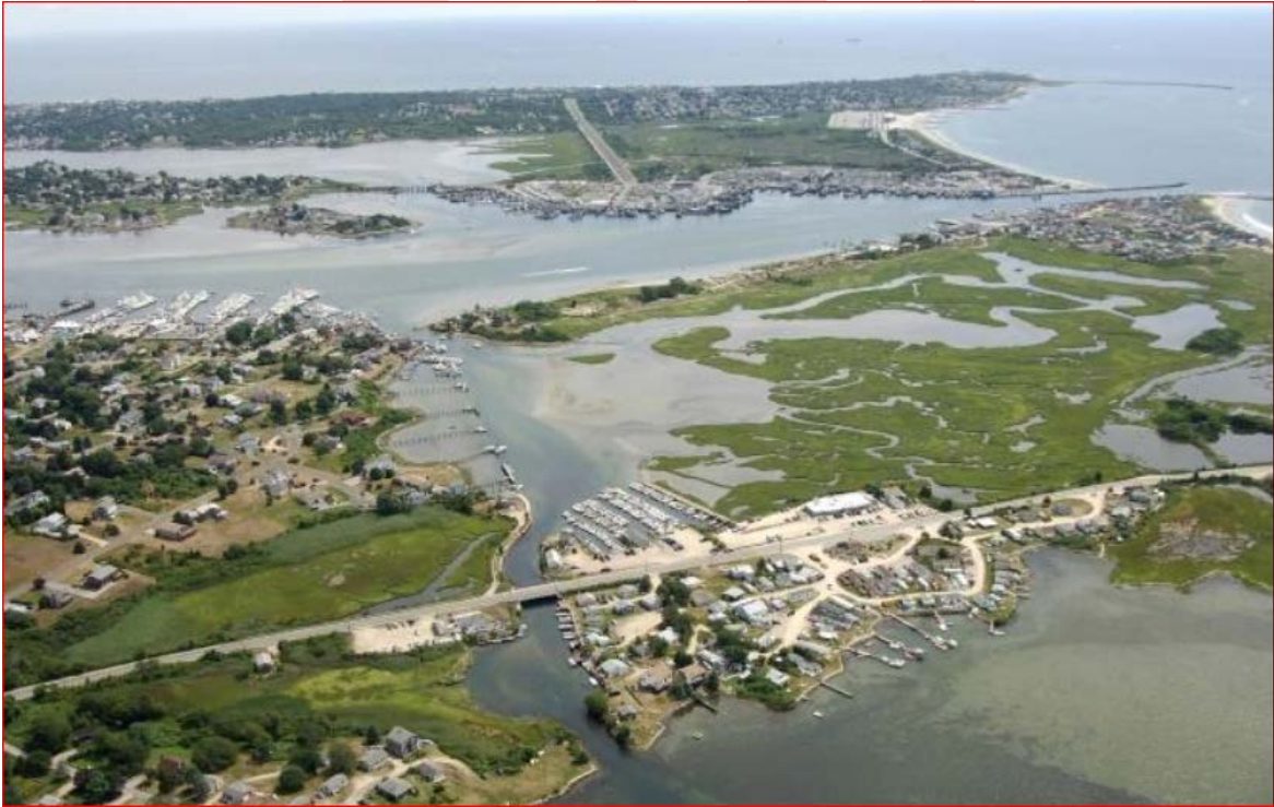
Figure 1-10. The inlet connecting Point Judith Pond and Potter Pond
