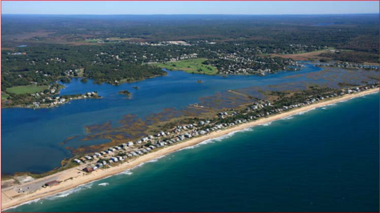
Figure 1-3. Middle area of Misquamicut constructed on barrier sand spit with backing marsh.
