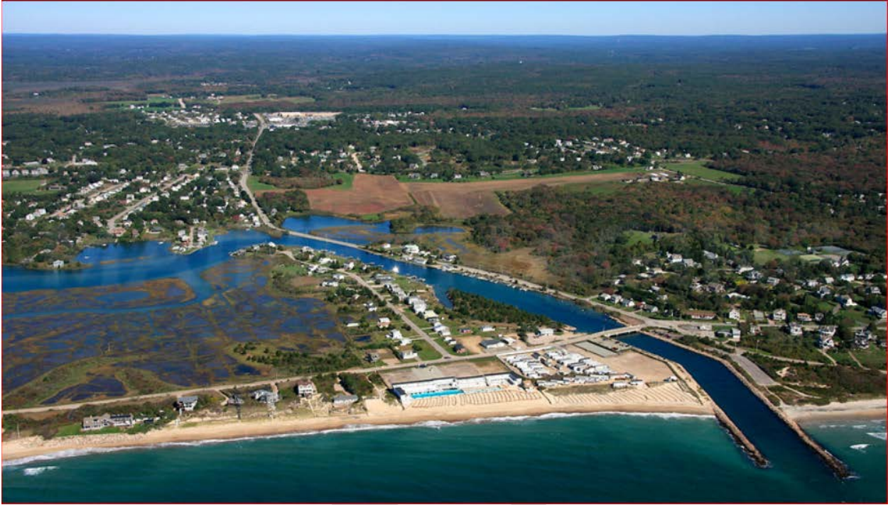
Figure 1-4. East end of Misquamicut and stabilized Winnapaug Pond inlet (Weekapaug Breachway)
