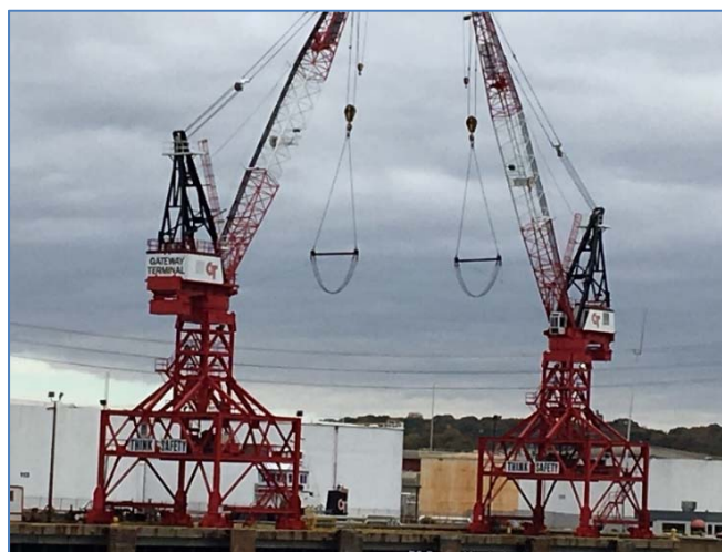
Figure 2-3c: Gateway Terminal Cranes
