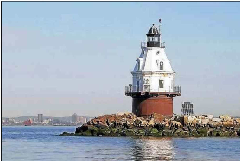
Figure 2-1: View of Lighthouse on East Breakwater
