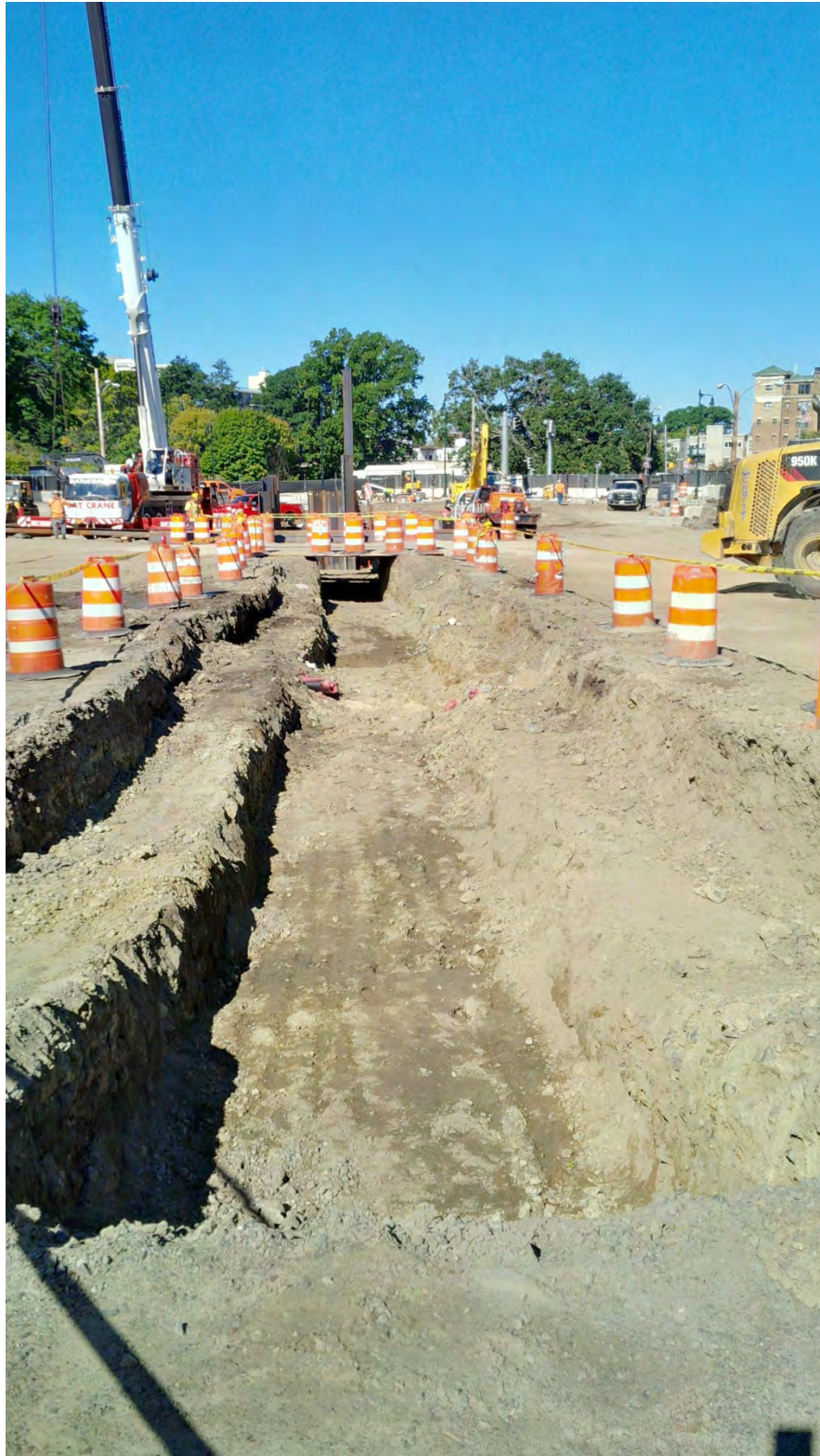
Pre-excavation in the former Sears Parking Lot for the river diversion steel sheeting line – note the removal of the temporary utilities line – early October 2015.
