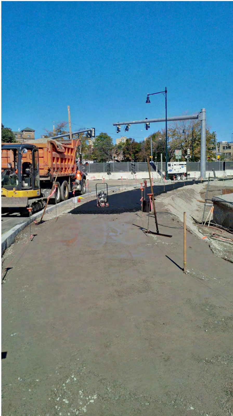
New pedestrian pathway over new Riverway Culvert – note the new traffic signal and new ornamental streetlight in the background – mid October 2015.
