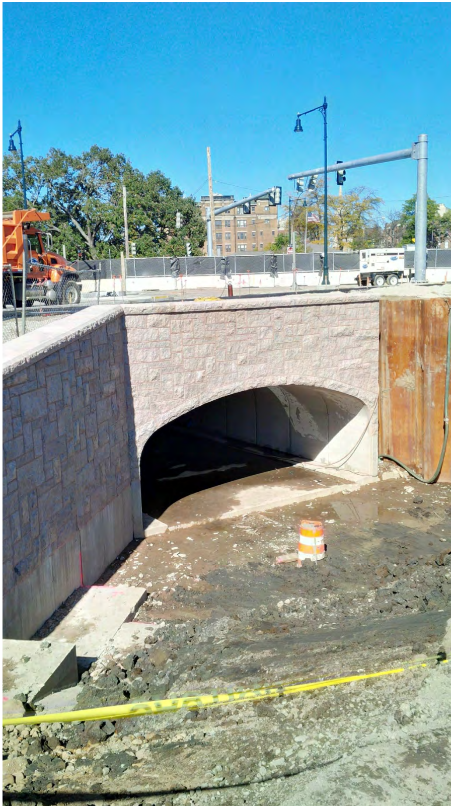
New Riverway Culvert in the former Sears Parking Lot – note the granite veneer installed on the precast culvert and the wingwall that cannot be completed until the existing twin 72" culverts are removed – mid October 2015.
