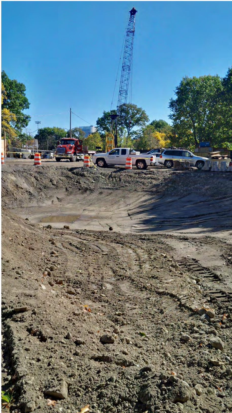
Excavation of the area between Upper Fens Pond and Avenue Louis Pasteur to daylight and begin construction of the Flood Risk Management Channel – mid October 2015.
