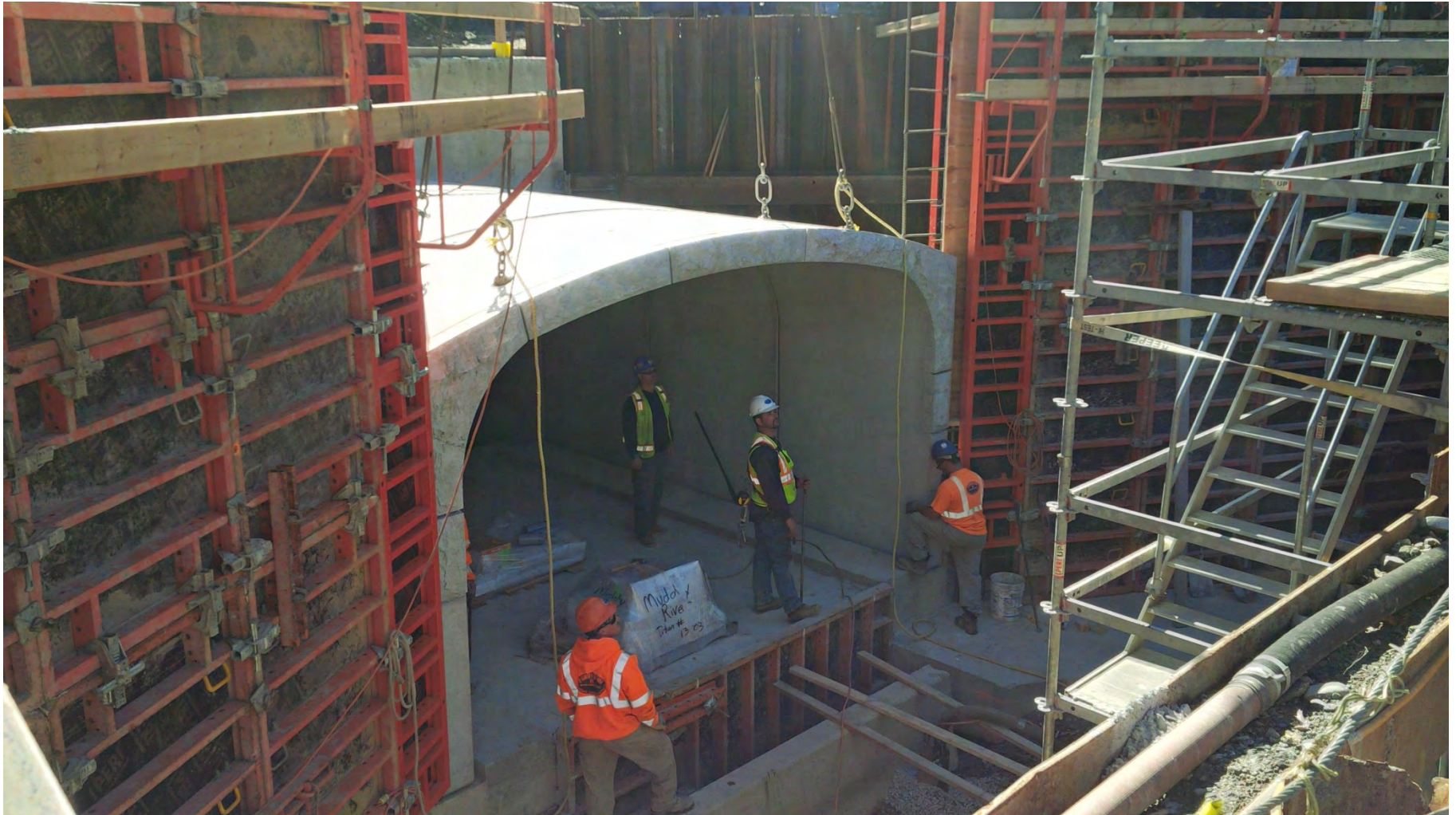
Precast concrete culvert section installed at the Avenue Louis Pasteur culvert – note the attached granite veneer on the culvert face and the formwork and rebar for the wingwalls on either side of the precast culvert – mid October 2015.
