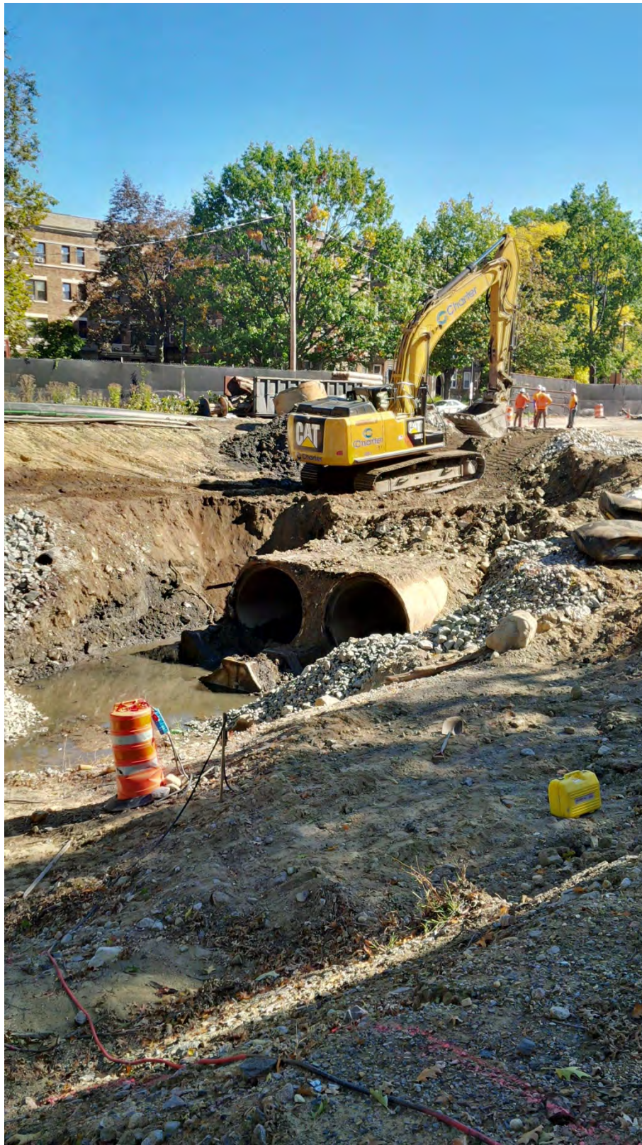
Downstream end of the Upper Fens Pond, where the existing twin 72" culverts begin – note that the excavation to daylight the area between Upper Fens Pond and Avenue Louis Pasteur has begun – mid October 2015.
