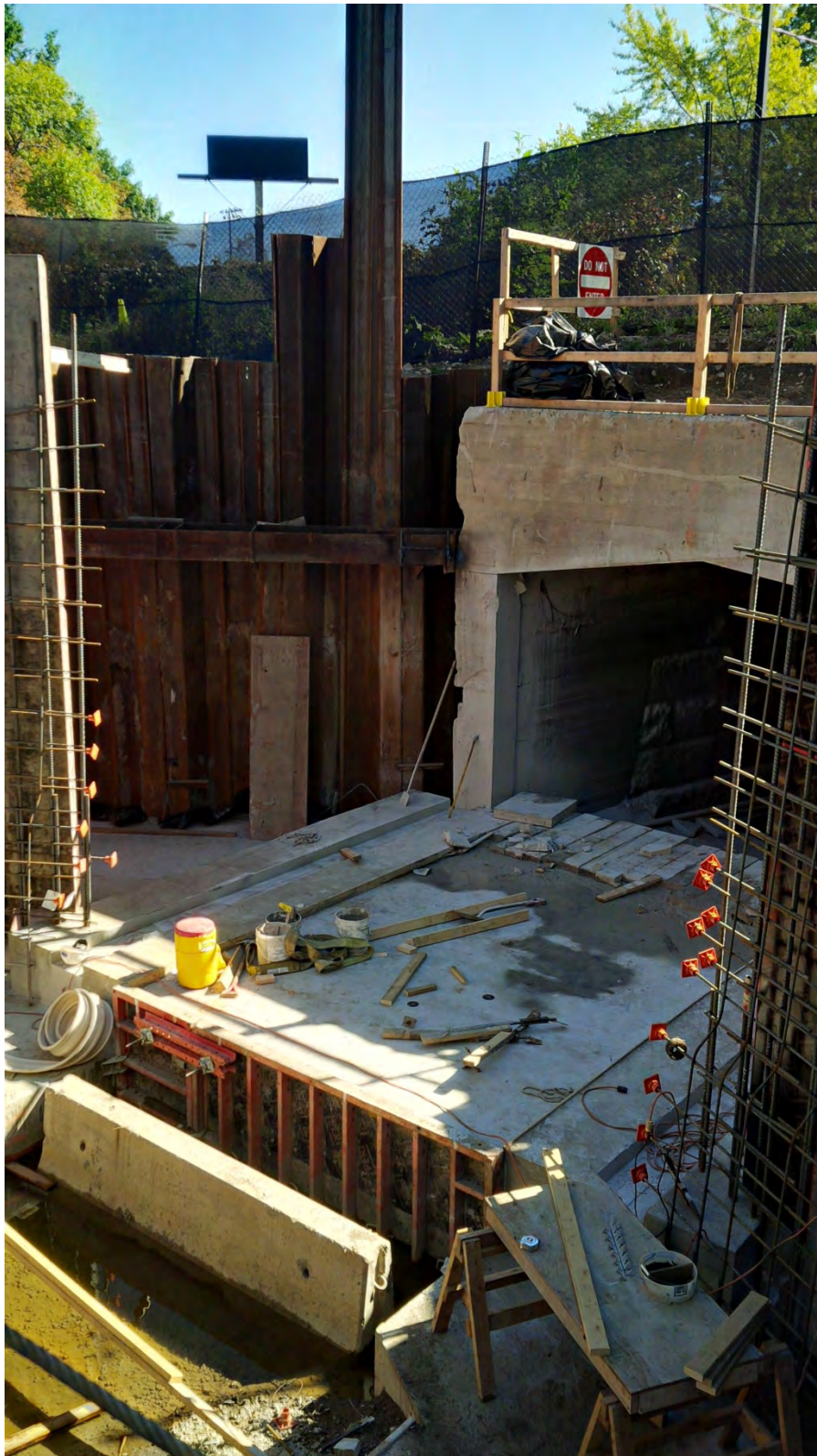
Existing concrete junction box of the Avenue Louis Pasteur culvert – note the new invert slab and the formwork and rebar for the wingwalls of the new precast concrete culvert extension – early October 2015.
