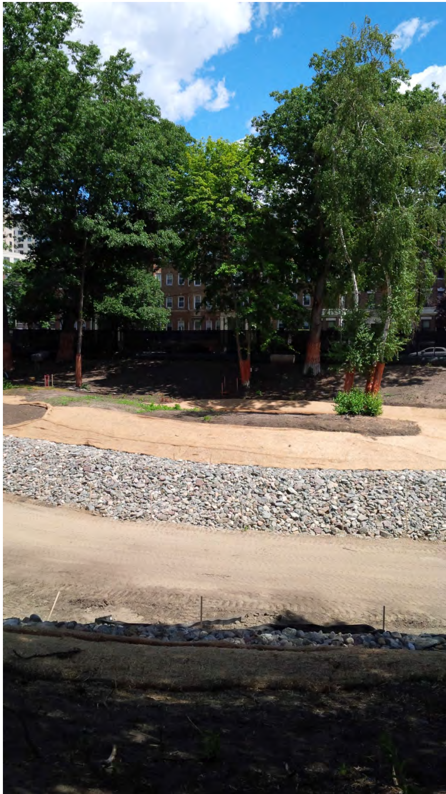
Completed bank protection/restoration at left bank of Upper Fens Pond – awaiting plantings in the Fall – late July 2015.
