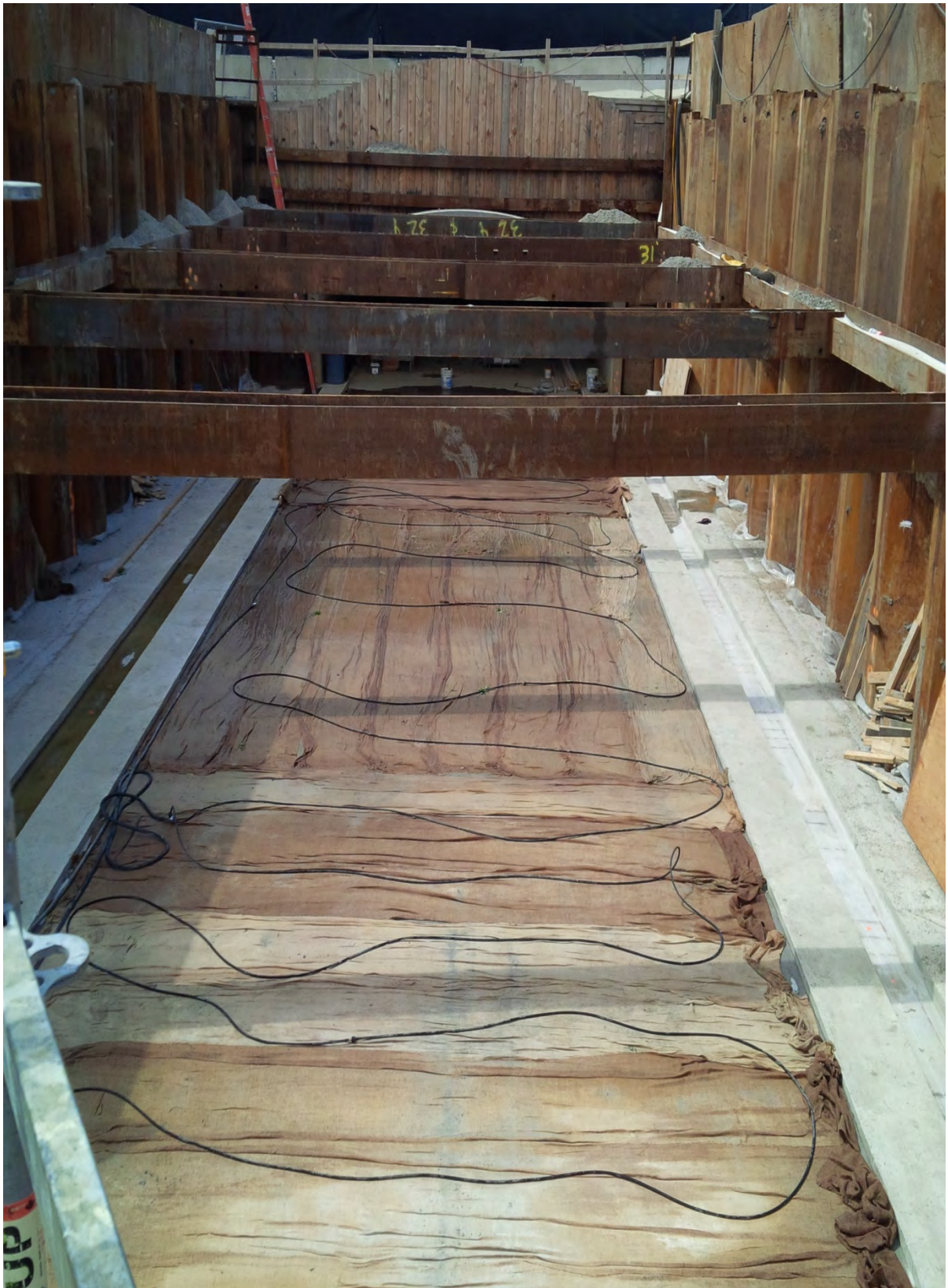
Forms for the pile caps stripped; and invert slab curing in advance of the new precast concrete Riverway Culvert placement – early August 2015.
