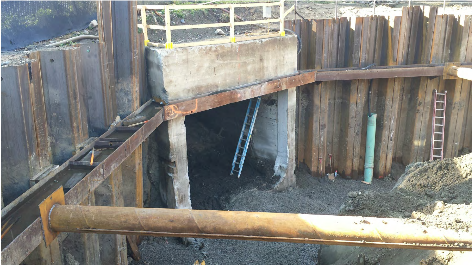
Upstream of Existing Avenue Louis Pasteur – existing twin 72" culverts removed and existing junction box cut open in preparation to receive the precast culvert extension pieces in early October – 12 August 2015.
