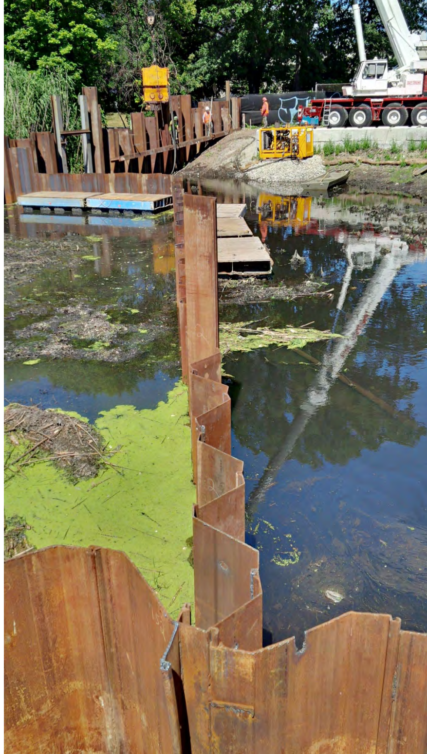
View of FRCS and the cofferdam that temporarily bisects the river – the cofferdam allows for the continued flow of the river on one side while sediment removal/bank restoration takes place on the other side – early August 2015.
