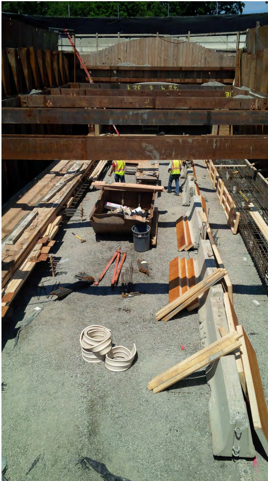
Right (looking downstream) concrete pile cap curing; and reinforcement and formwork being installed at the left pile cap for the new precast concrete Riverway Culvert – mid July 2015.
