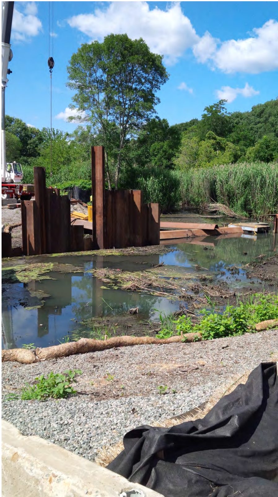
Upstream limits of Phase 1 Construction – line of steel sheeting is the installed Flow Restriction Control Structure (FRCS) – about 100' upstream of the existing Riverway Intake Structure – end July 2015.
