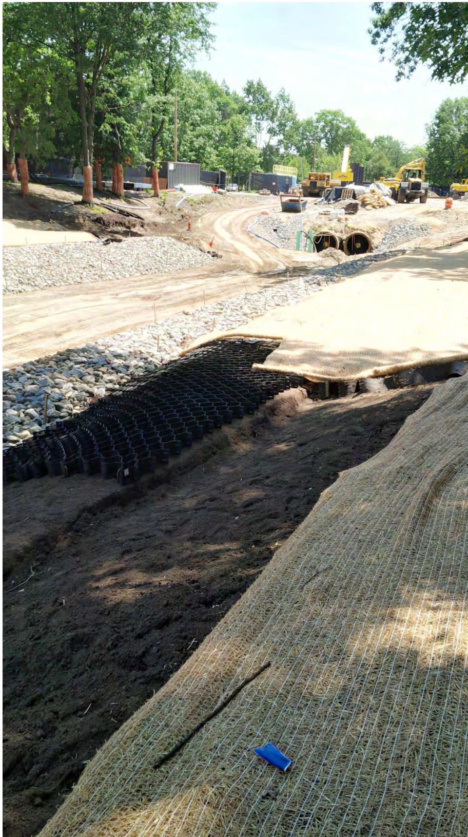
Bank stabilization/construction with stone protection; geocells; loam; and turf reinforcement mattress at Upper Fens Pond. Note the existing twin 72" culverts that will be removed as part of the daylighting to connect the Upper Fens Pond to Avenue Louis Pasteur – mid July 2015.
