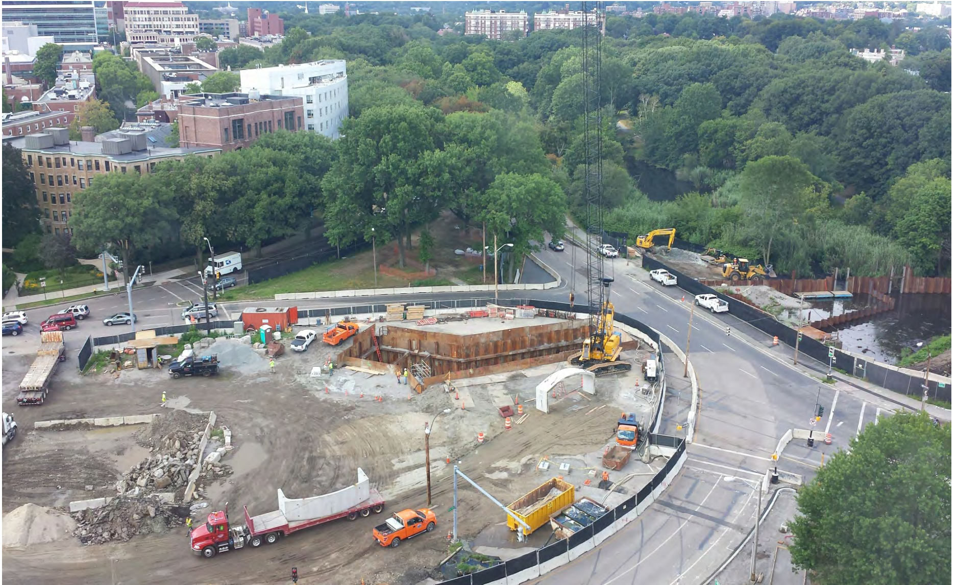
Aerial photo of the former Sears Parking Lot – Note the crane is lifting the Riverway precast concrete culverts into place – 12 August 2015.
