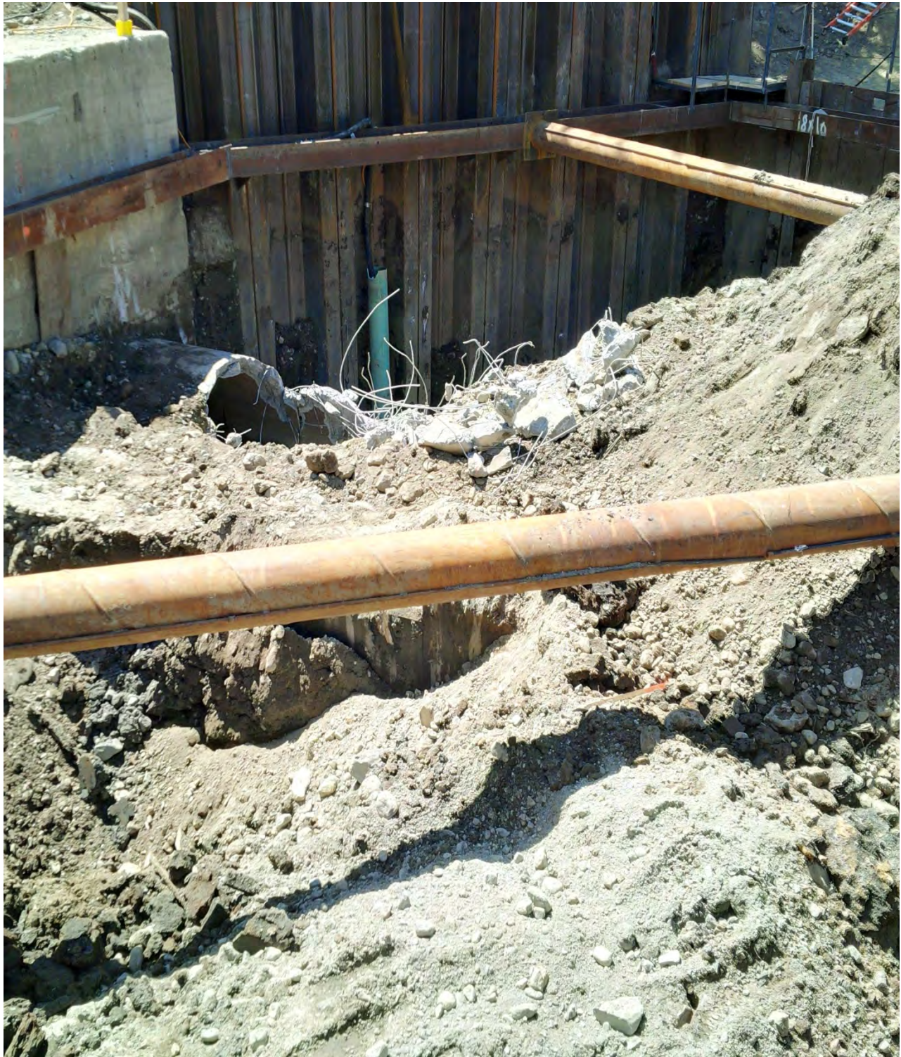
Upstream of Existing Avenue Louis Pasteur – Support of excavation installed; excavation of hole has begun; one of the existing 72" culverts selectively demolished to investigate its condition – early August 2015.
