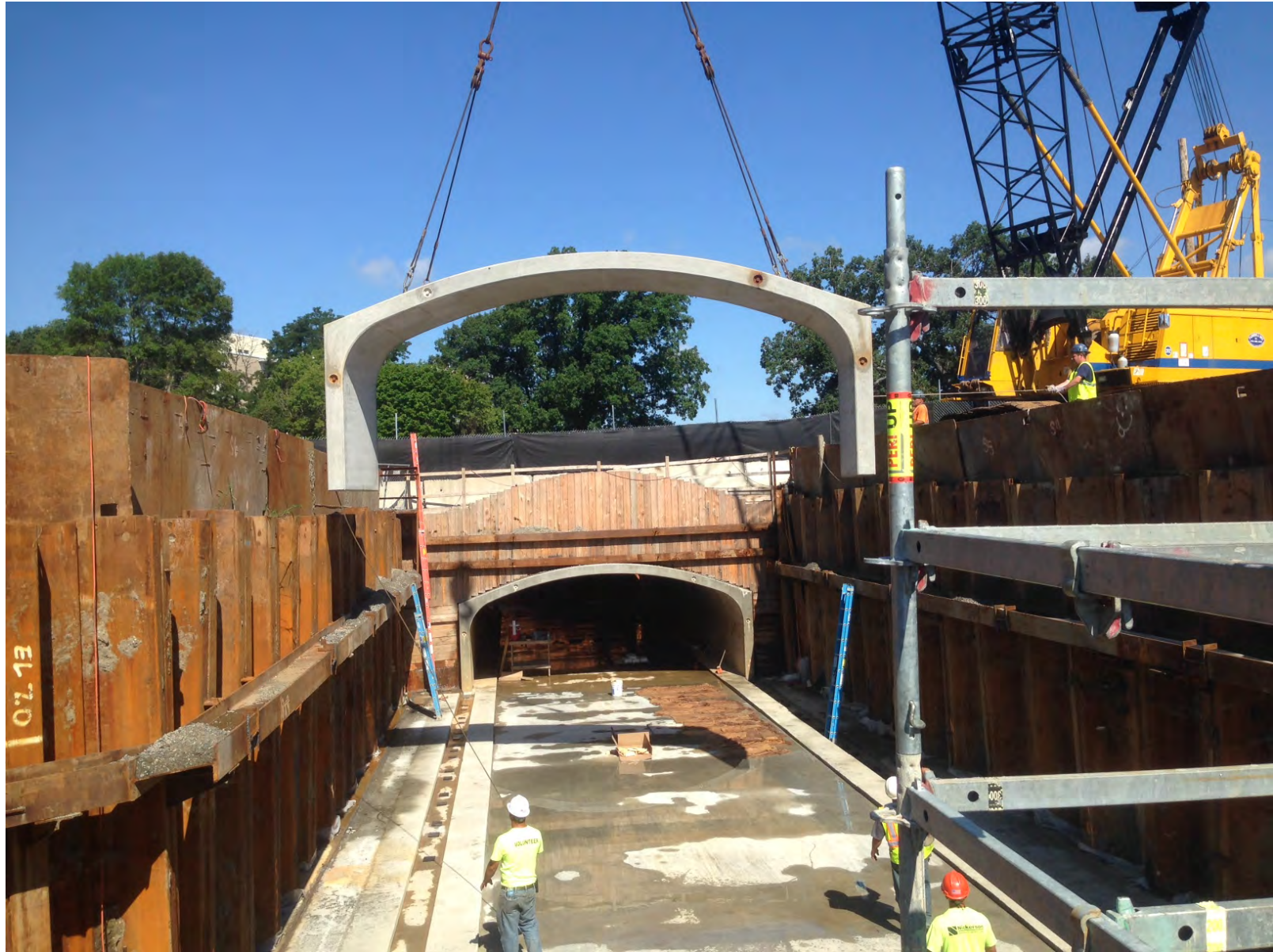
Precast concrete culvert section being placed for the new Riverway Culvert – 12 August 2015.
