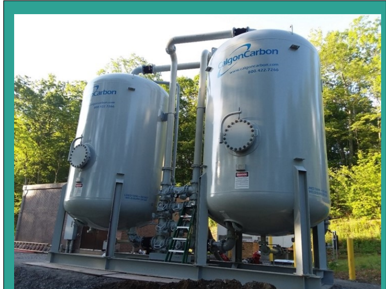
Two 20,000-pound carbon units treat water from the Grove Pond wellfield.
