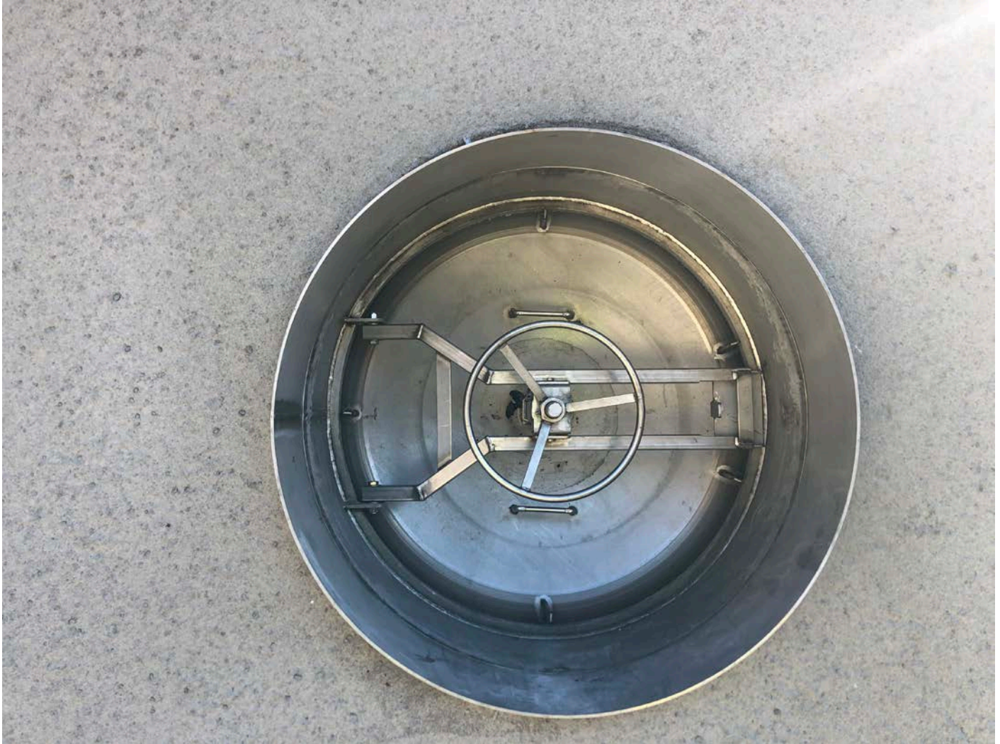
Picture 6: Tank hatch installed on the west side of the water tank that is located to the east of the Shared Access Driveway, Middletown. View to the east.
