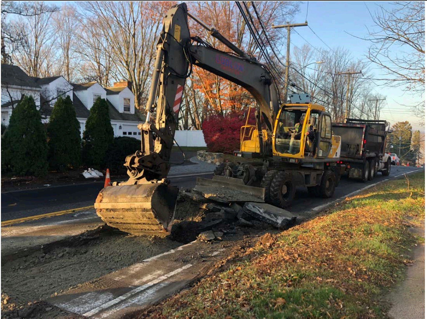
Picture 2: Ludlow stripping pavement from trench overcuts on the westbound lane of Route 68, Durham as part of permanent paving activities. View to the southwest.
