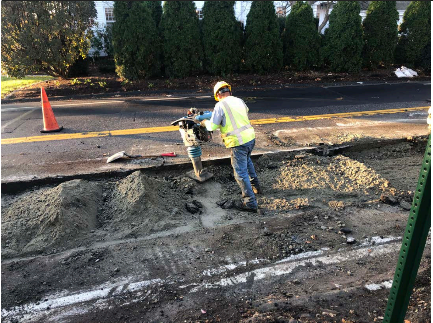
Picture 1: Ludlow compacting 1.5" gravel at Station 601+00 on the westbound lane of Route 68, Durham as part of permanent paving activities. View to the south.
