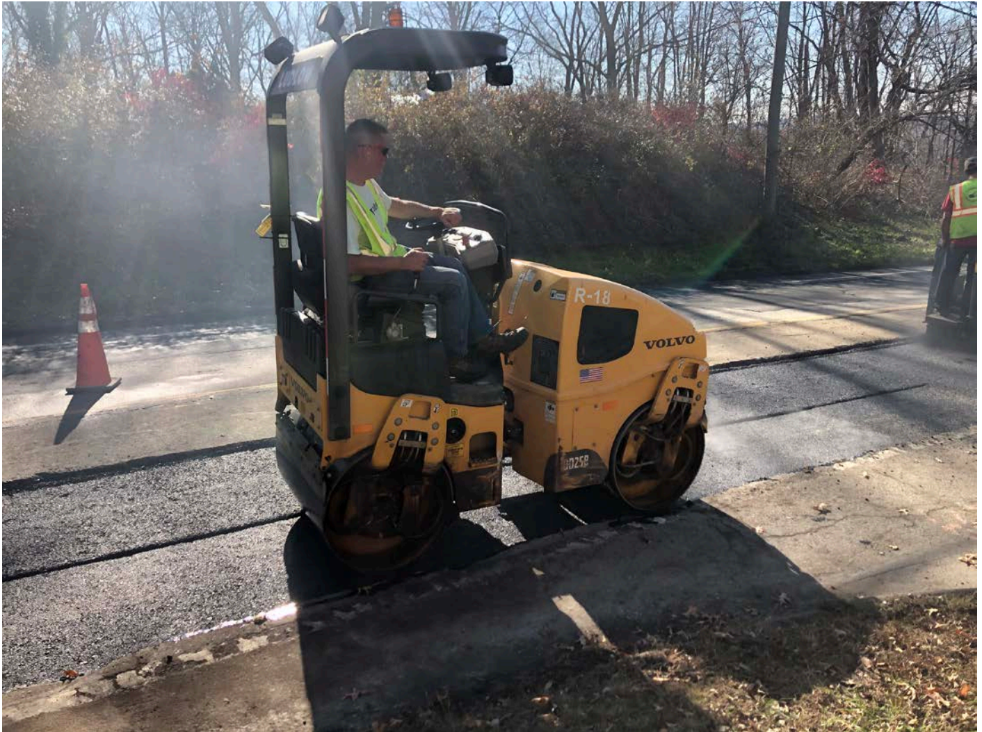
Picture 8: Ludlow compacting the second of three 3” lifts of asphalt as part of permanent paving activities on the westbound lane of Route 68, Durham as part of permanent paving activities. View to the southwest.
