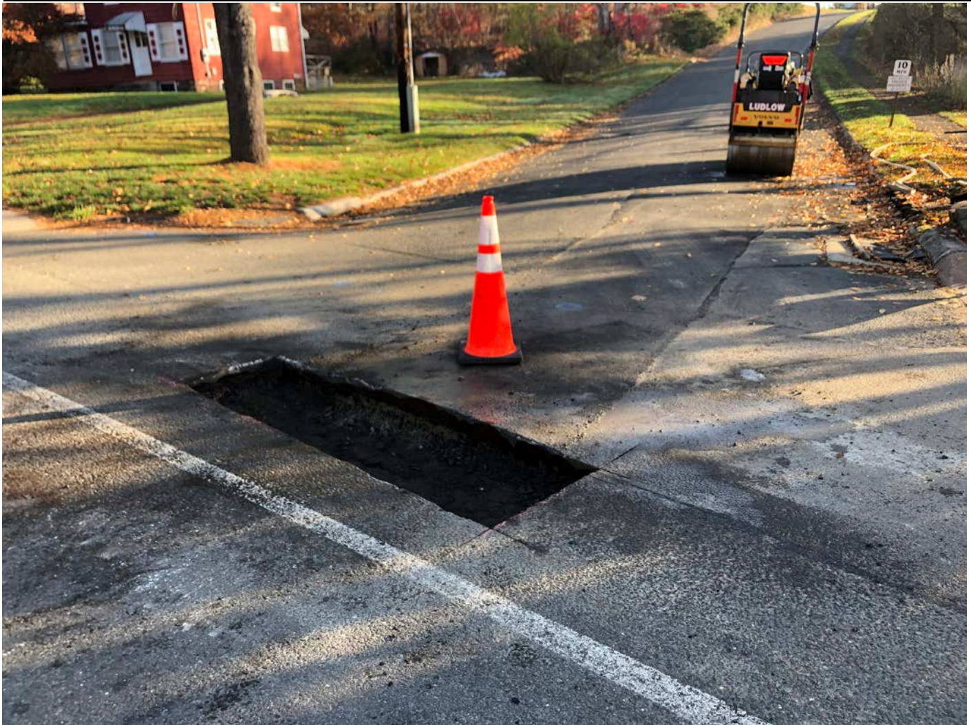
Picture 3: Pavement Ludlow excavated at the intersection of Mill Pond Lane and Main Street, Durham Station 209+51 as part of permanent paving activities on the northbound lane of Main Street, Durham. View to the northeast.
