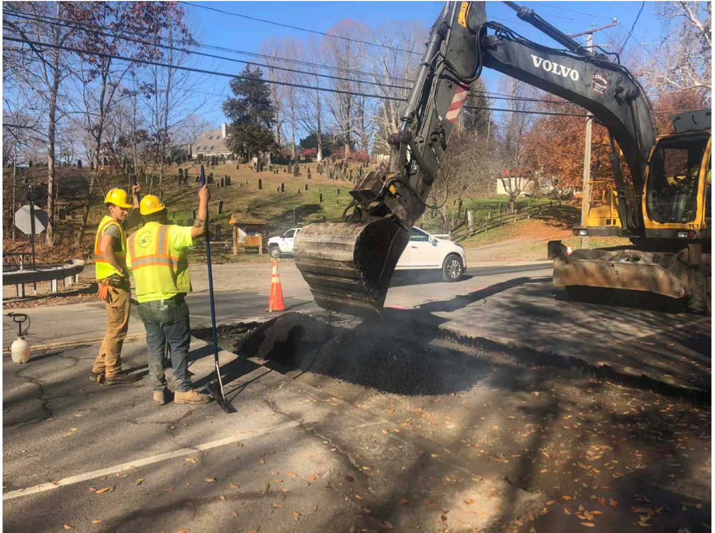
Picture 5: Ludlow placing the first of three 3” lifts of asphalt at the curb stop overcut located at Station 209+55 on the northbound lane of Main Street, Durham. View to the northwest.
