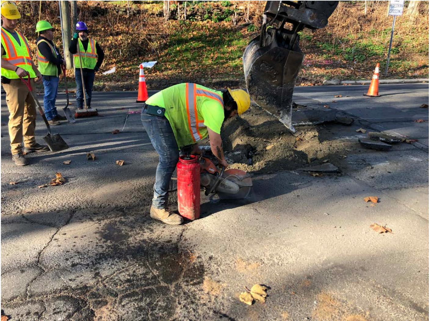
Picture 4: Ludlow saw cutting pavement at the intersection of Pickett Lane and the northbound lane of Main Street, Durham as part of permanent paving activities. View to the west.
