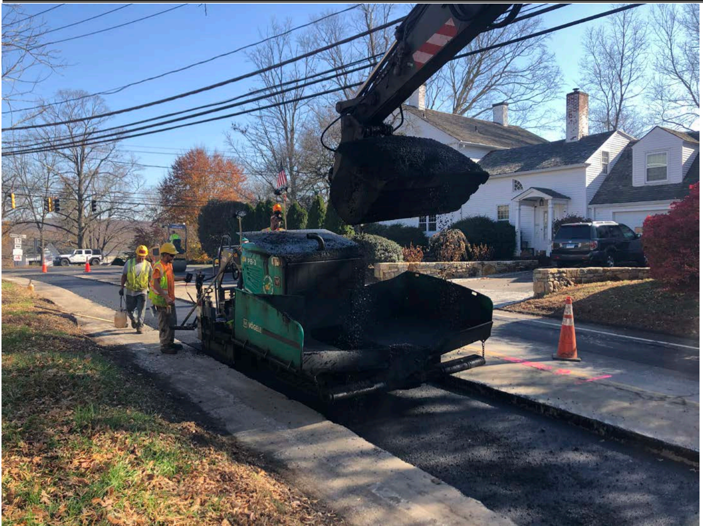
Picture 7: Ludlow placing the second of three 3" lifts of asphalt as part of permanent paving activities on the westbound lane of Route 68, Durham as part of permanent paving activities. View to the southeast.
