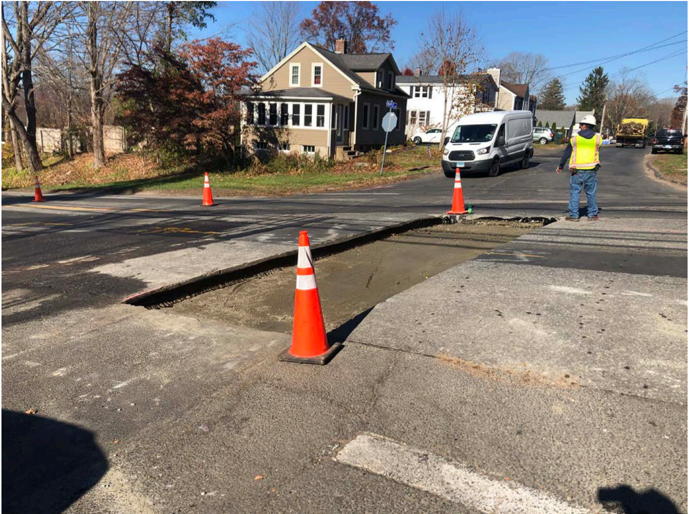
Picture 7: Trench overcut that Ludlow excavated as part of permanent paving activities on the eastbound lane of Route 68, Durham where it intersects with Maple Avenue, Durham at Station 606+65.
