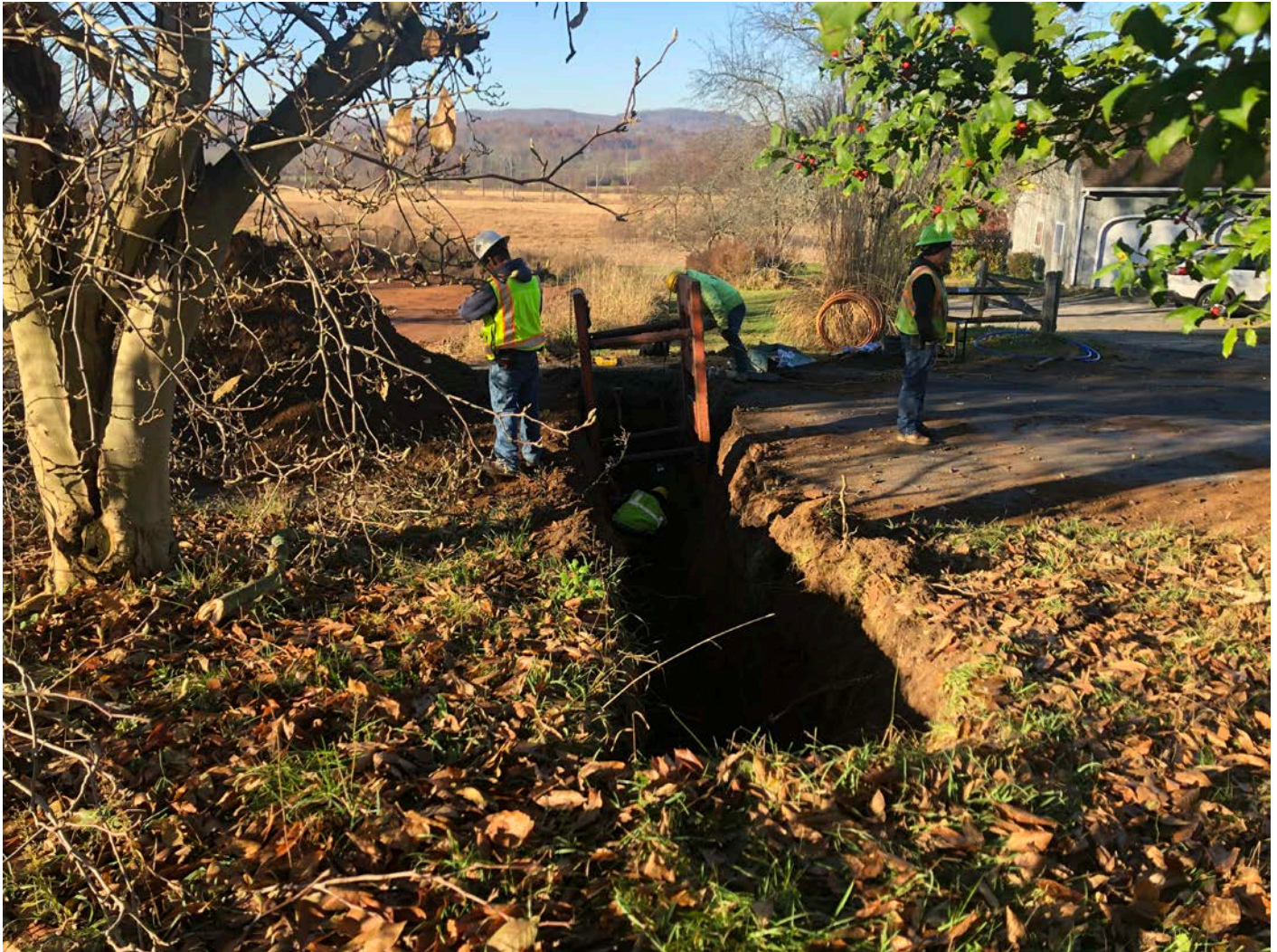
Picture 2: Ludlow installing a curb stop for the empty lot located adjacent to, and immediately north of, 133 Maple Avenue, Durham at Station 917+60. View to the west.
