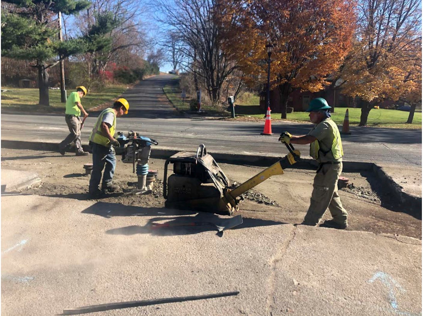
Picture 6: Ludlow compacting 1.5" processed gravel as part of permanent paving activities between Stations 207+90 and 209+41 on the southbound lane of Main Street, Durham. View to the east.
