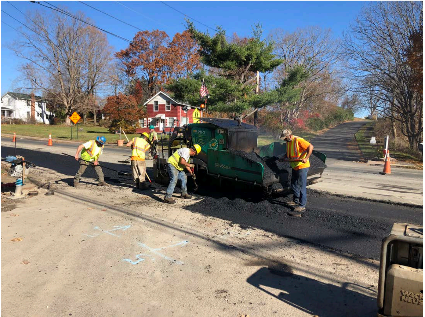
Picture 9: Ludlow placing the third of three 3" lifts of asphalt as part of permanent paving activities between Stations 207+90 and 209+41 on the southbound lane of Main Street, Durham. View to the northeast.
