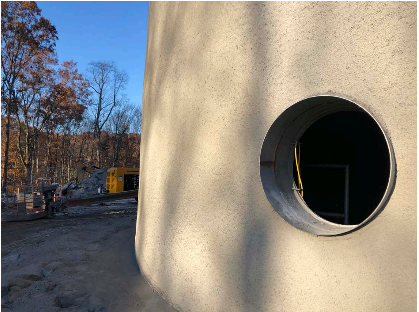
Picture 1: Manway on the east side of the water tank located to the east of the Shared Access Driveway, Middletown. View to the west.
