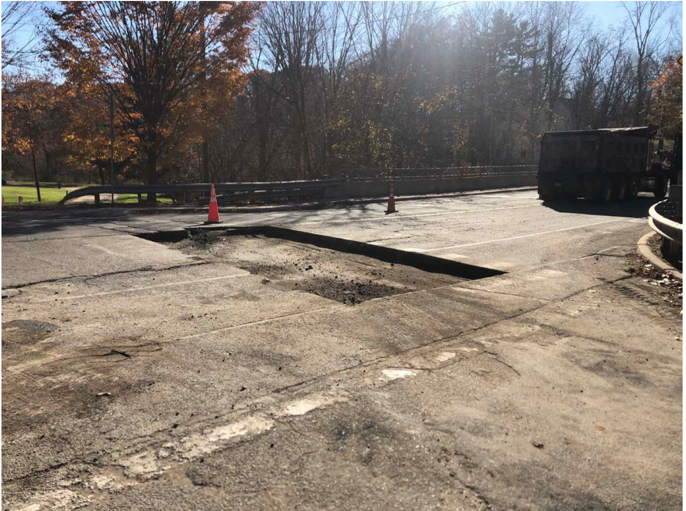
Picture 3: Curb stop overcut located at Station 209+51 that Ludlow excavated as part of permanent paving activities on the northbound lane of Main Street, Durham. View to the southeast.
