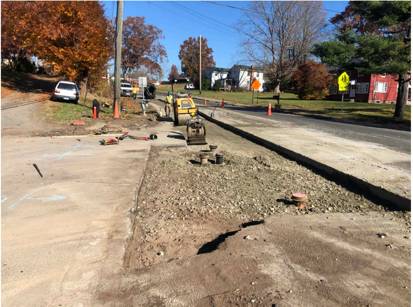
Picture 4: Pavement stripped from trench overcuts between Stations 207+90 and 209+41 on the southbound lane of Main Street, Durham as part of permanent paving activities. View to the north.
