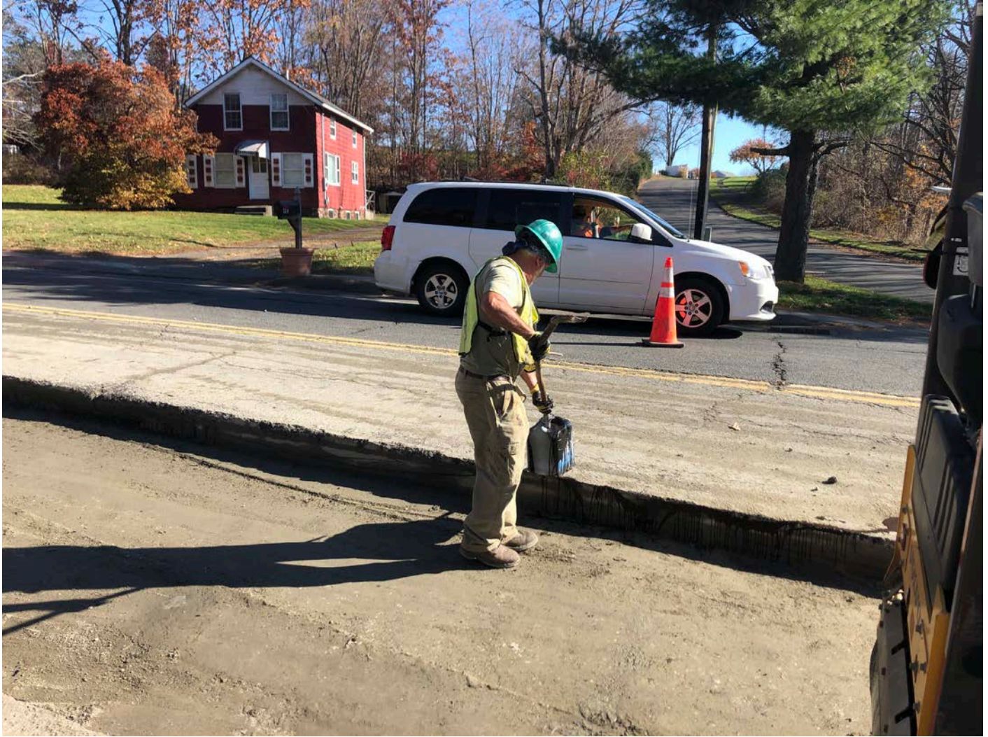
Picture 5: Ludlow apply tack coat to the edges of cut pavement as part of permanent paving activities between Stations 207+90 and 209+41 on the southbound lane of Main Street, Durham. View to the east.
