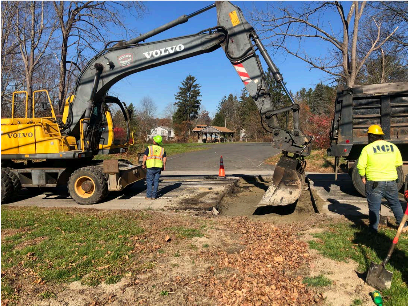
Picture 8: Ludlow placing and compacting 1.5” processed gravel at the curb stop overcut located at Station 604+61 on the eastbound lane of Route 68, Durham as part of permanent paving activities. View to the north.
