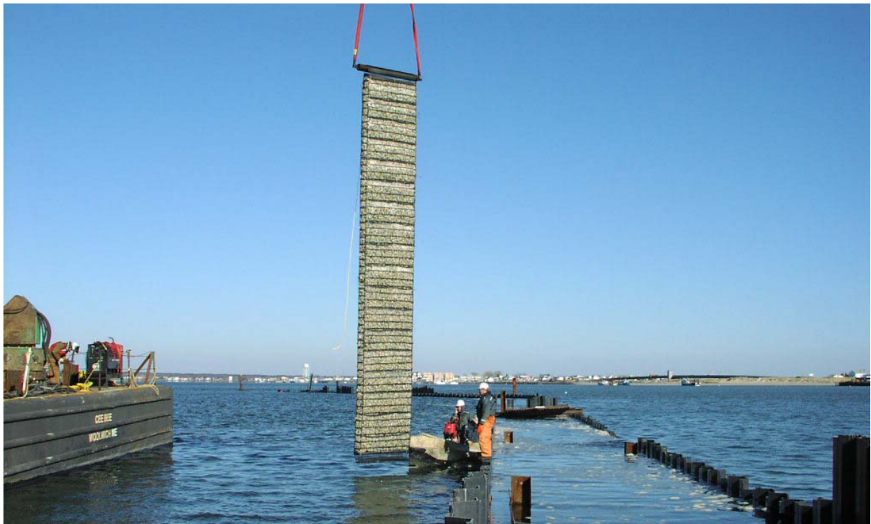
Photo 4 – Hoisting filled mattress for placement
