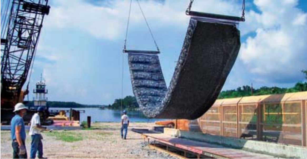
Photo 6 – Geotextile fabric attached to bottom of mattress
