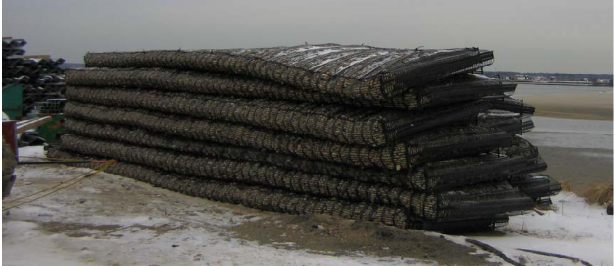
Photo 5 – Completed mattresses stacked prior to being placed
