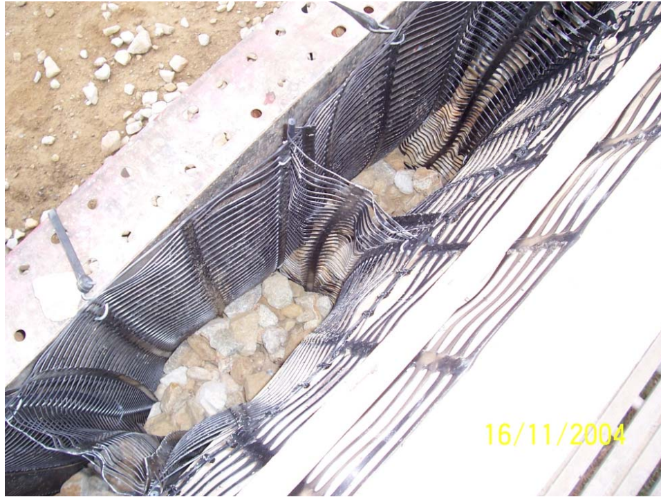
Photo 3 – View from top of form showing internal web structure of mattress
