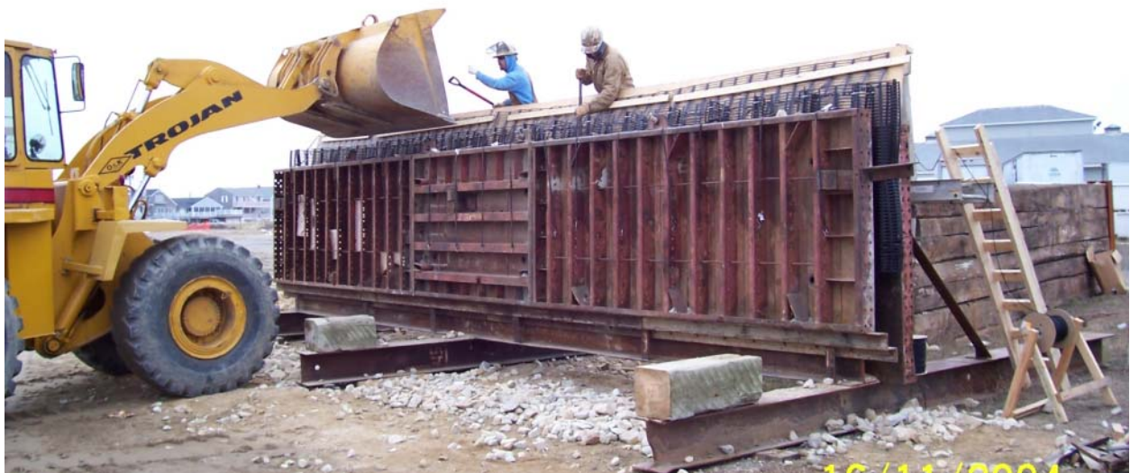
Photo 2 – Form used to fill mattresses on land
