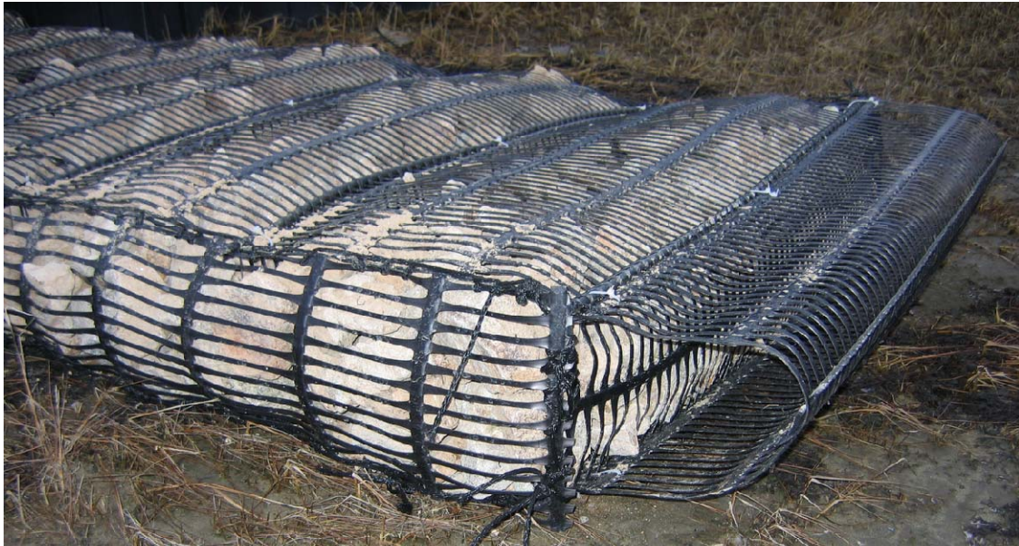
Photo 1 – Closeup of filled mattress
