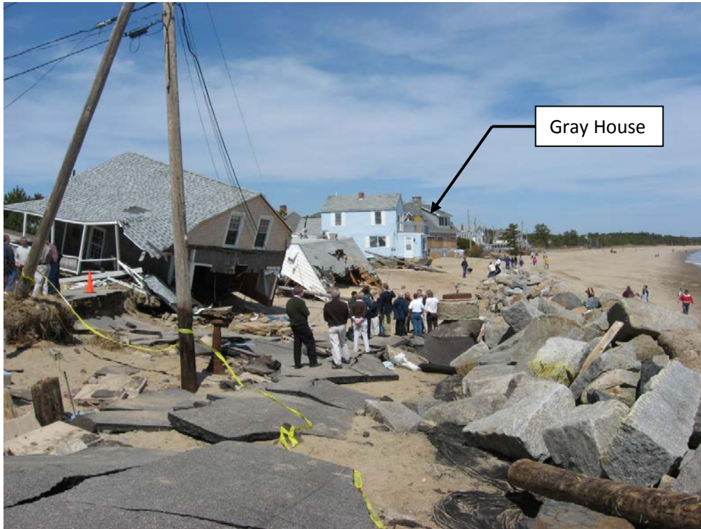
Figure 4-10. North end looking north - post storm April 2007. Destroyed road, houses and utilities and damaged revetment.
