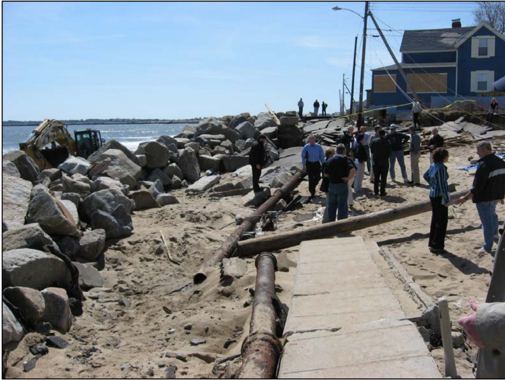
Figure 1-8. Damage at northern end to road, houses, utilities, and revetment (looking south).
