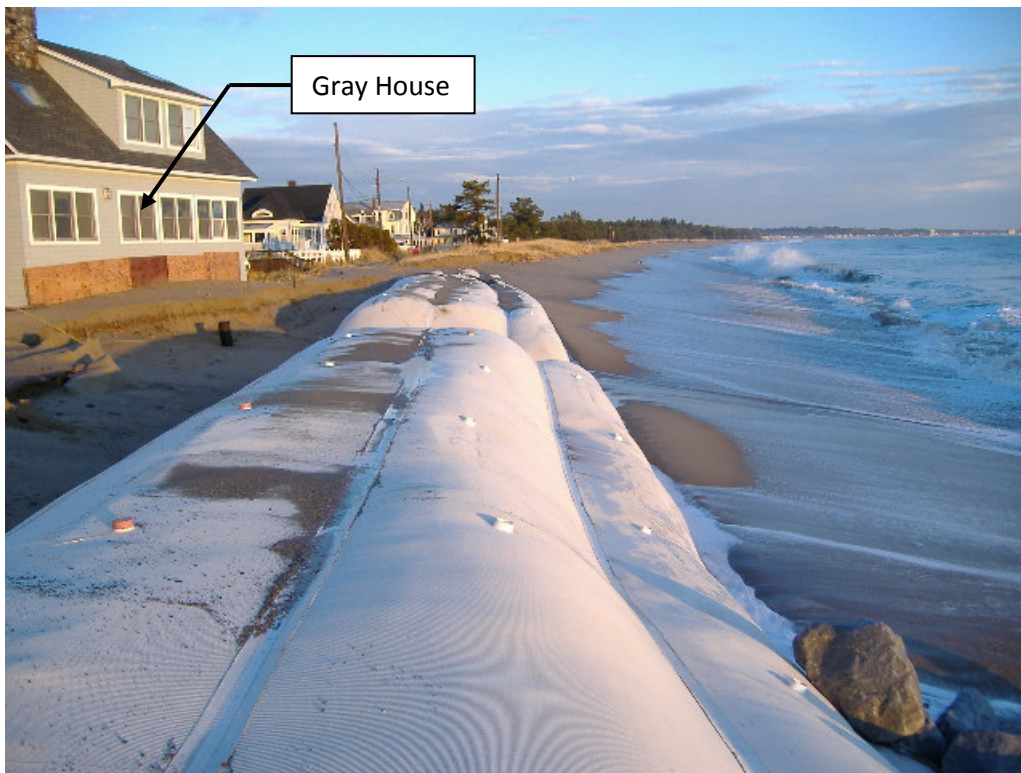
Figure 4-11. North end of project looking north (2010) - geotubes in place, the road is lost, trees are lost, dune is eroded.
