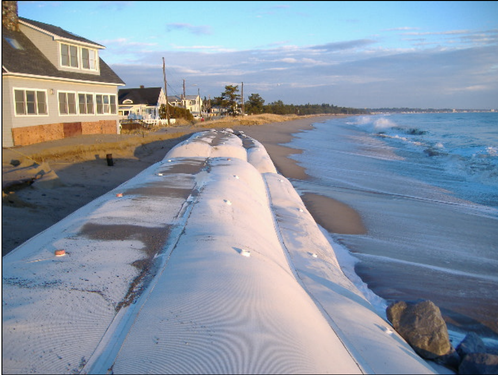
Figure 1-9. North end of project with geotubes placed at the end of the “temporary” revetments.
