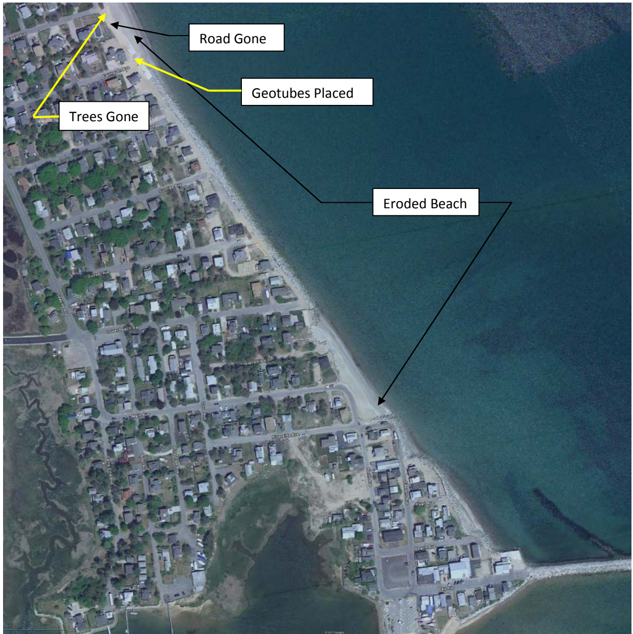
Figure 4-5. Google Earth Aerial Photo 2010 – Post-changes highlighted.
