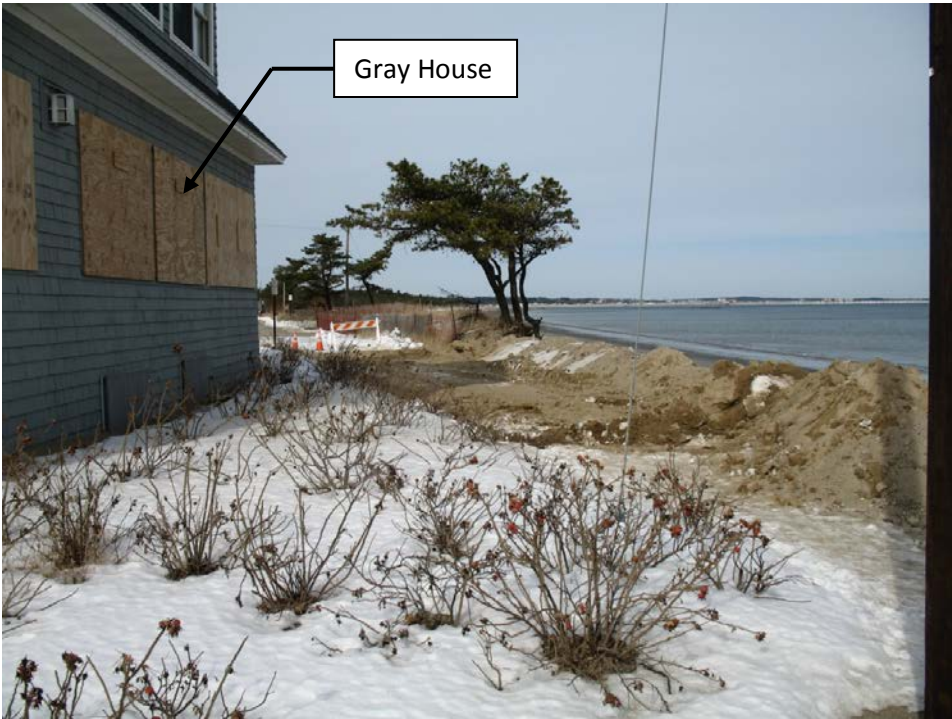
Figure 4-9. North end of the project – road lost (February 2007).
