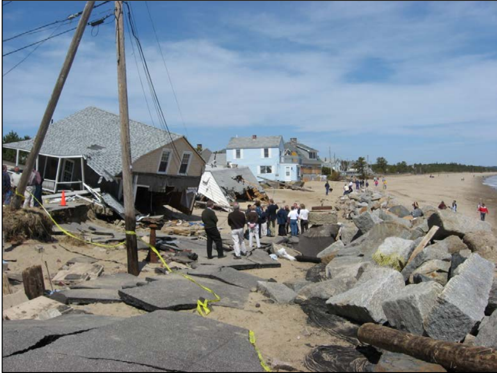
Figure 1-7. Damage at northern end to road, houses, utilities, and revetment (looking north).
