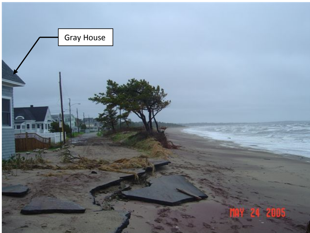
Figure 4-7. North end of the project looking north following a storm – road is damaged.
