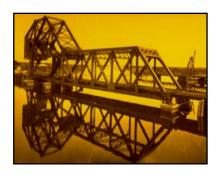
The 160-foot span pivoted on the north side of the Canal utilizing a single counterweight. The bridge in the raised position had an opening of 140 feet for vessels passing through. Two tracks crossed the bridge, one heading towards Provincetown and the other towards Woods Hole.
