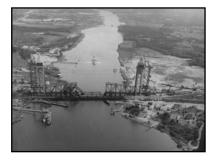
The railroad bridge was sited within 60 feet of the original in order to minimize the amount of track realignment.
