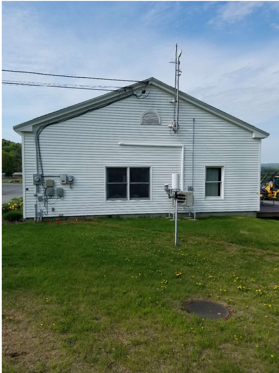
Informational Photo 3- Commercial power feed entrance
