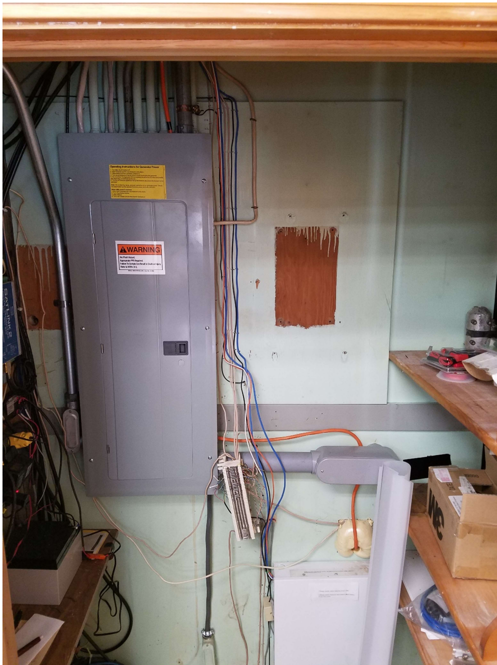
Informational Photo 2- Commercial power feed/200 amp panel and proposed automatic transfer switch location
