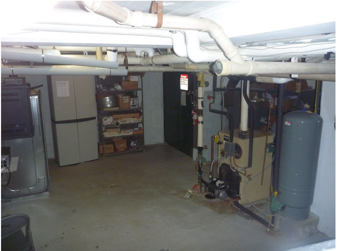
Informational Photo Number 2: Existing Oil Fired Boiler, Hot Water Tank and Oil Tank layout
