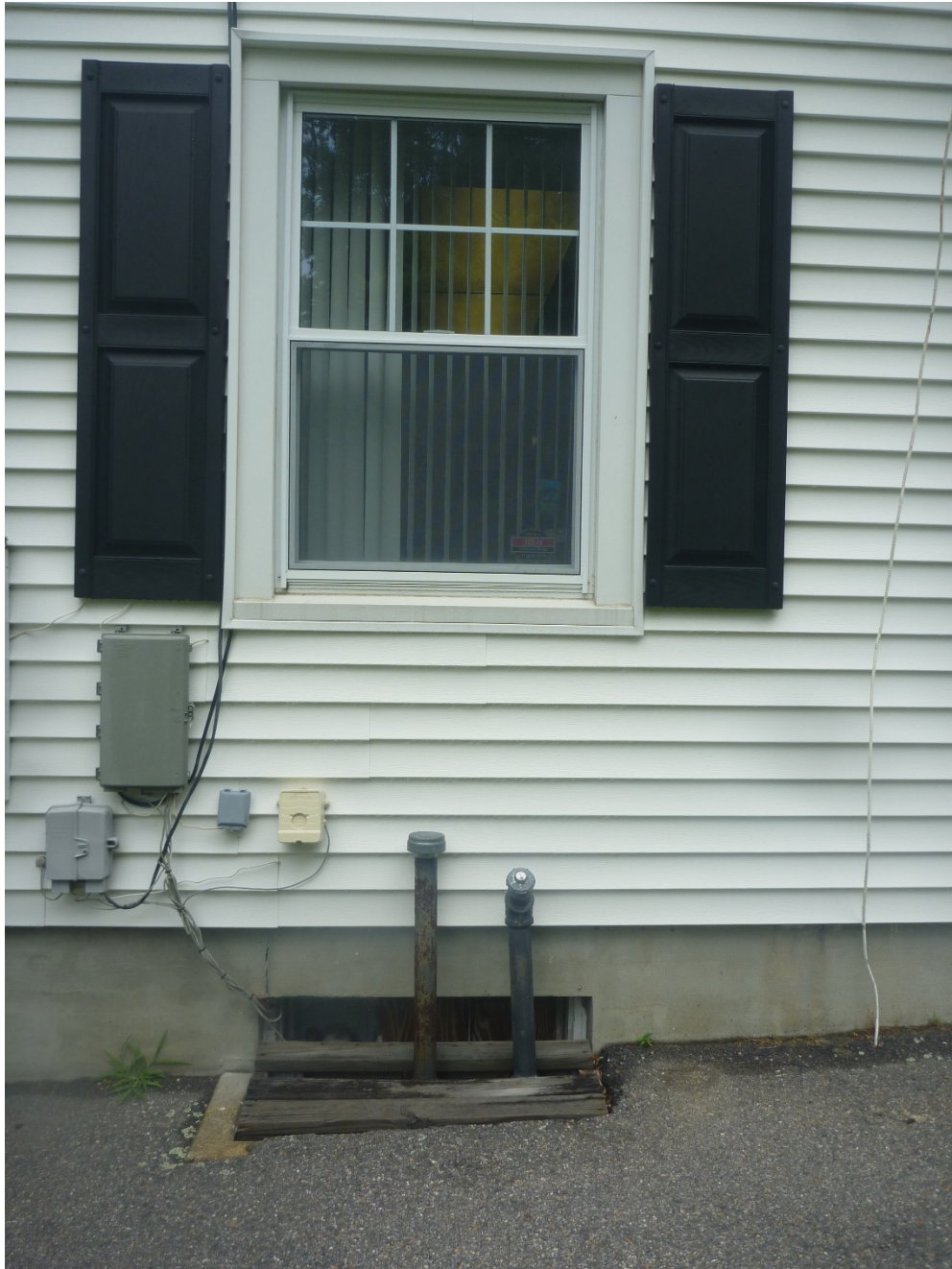
Informational Photo Number 6: Existing oil fill-up (basement window access) with nearby communication wiring.
