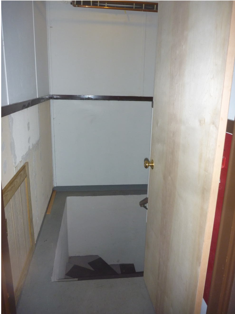
Informational Photo Number 5: 32" Doorway, Basement Stairwell Access
