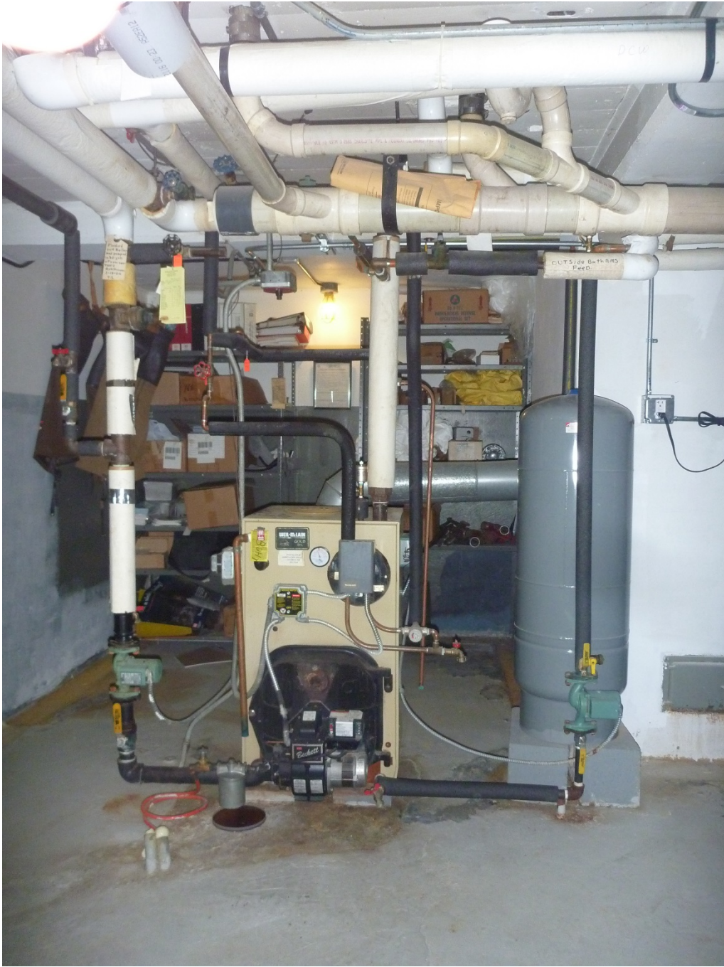
Informational Photo Number 3: Existing Oil Fired Boiler, hot water tank and heat zone piping (2 circulator pumps).
