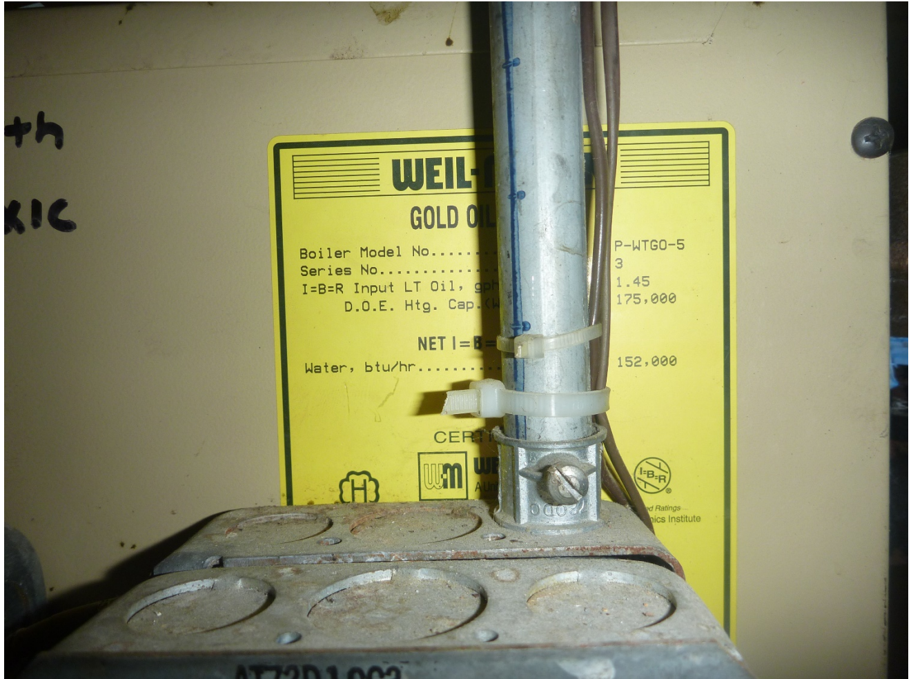
Informational Photo Number 1: Existing Oil Fired Boiler Manufacture's Plate
