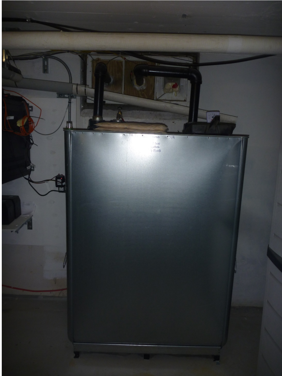
Information Photo Number 4: Existing oil tank and basement window used for fill-up access.
