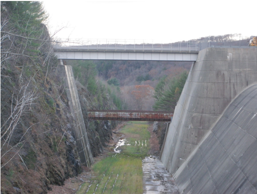
Photo 24: Thomaston Dam Spillway Bridge – Elevation View
