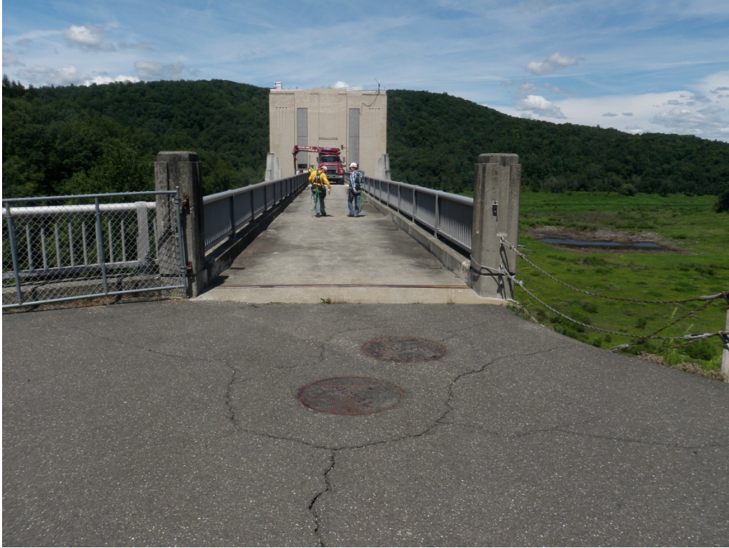
Photo 15: Knightville Dam Service Bridge – Plan View
