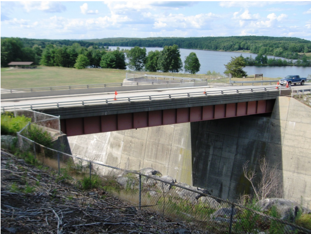
Photo 22: W. Thompson Lake Spillway Bridge – Elevation View
