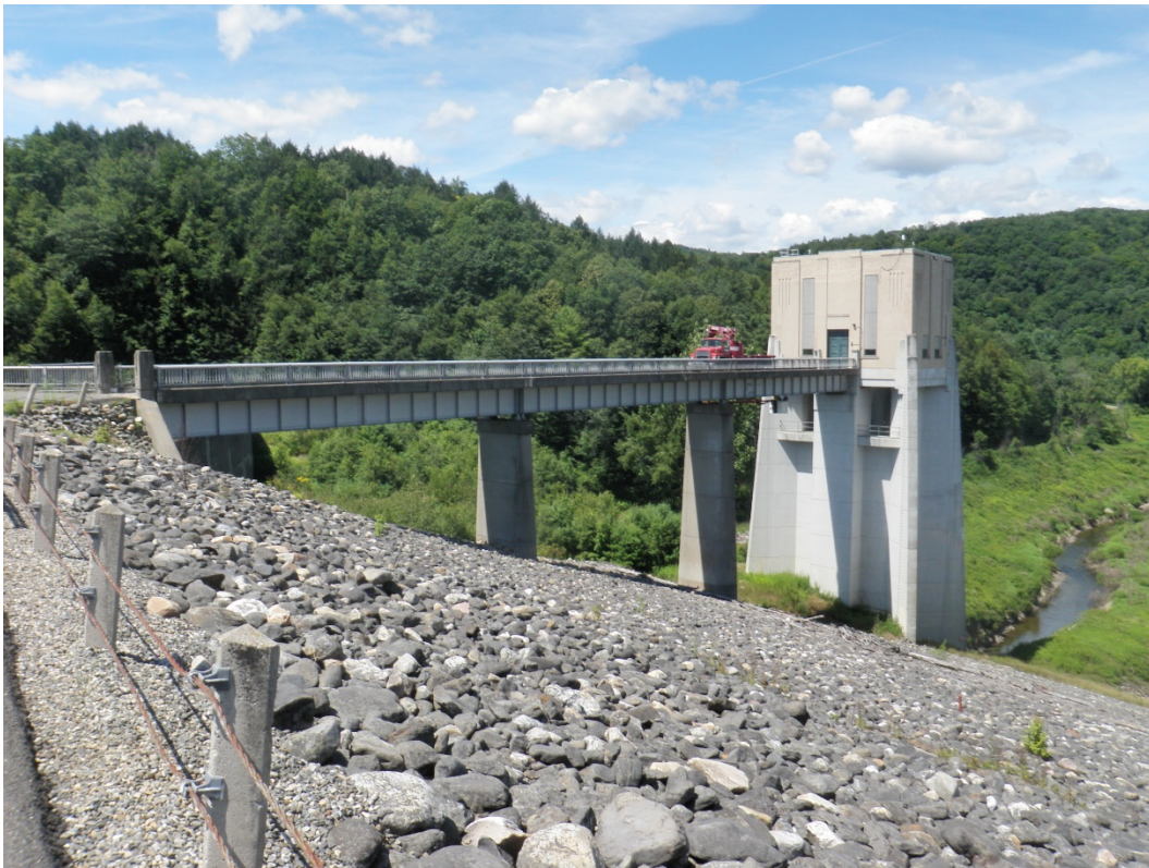
Photo 16: Knightville Dam Service Bridge – Elevation View
