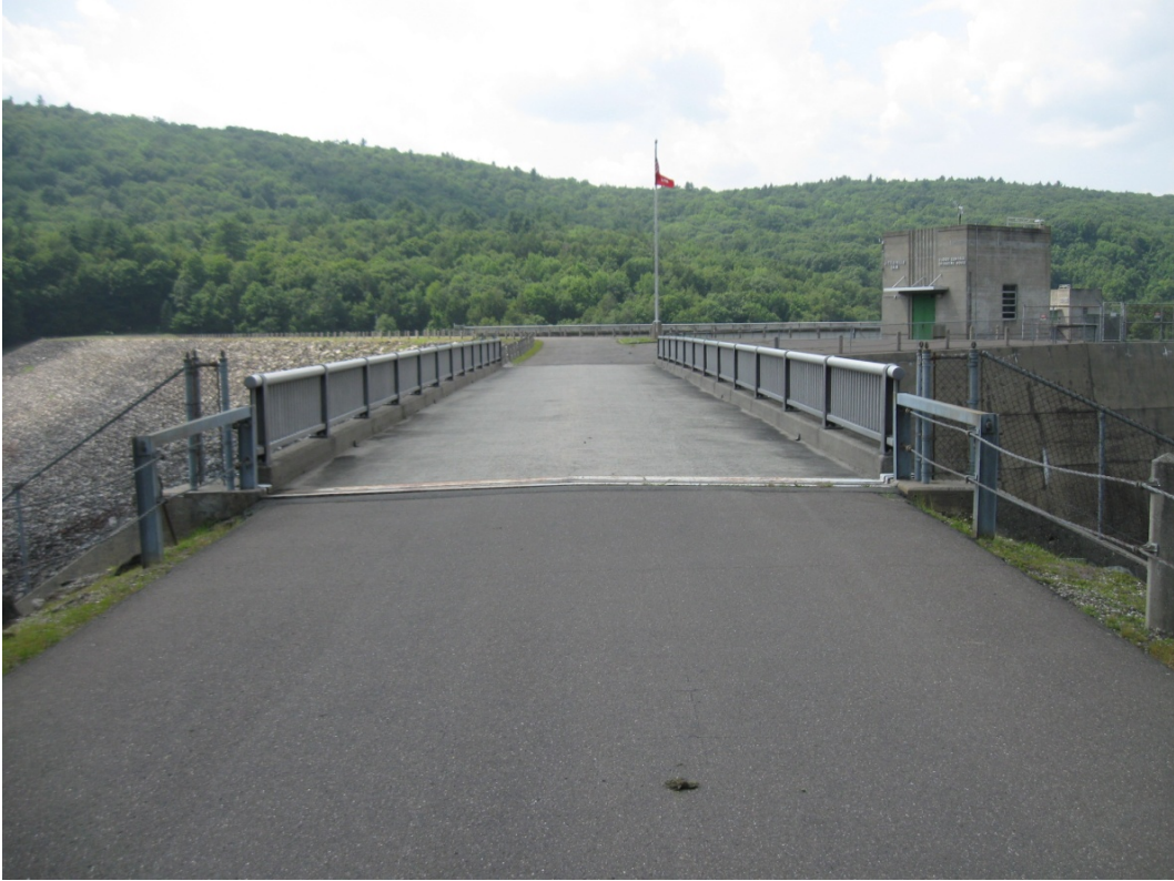
Photo 19: Littleville Lake Spillway Bridge – Plan View
