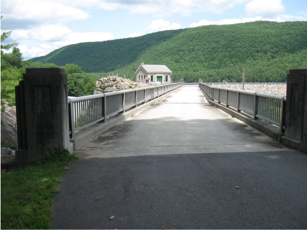
Photo 5: Surry Mountain Lake Spillway Bridge – Plan View
