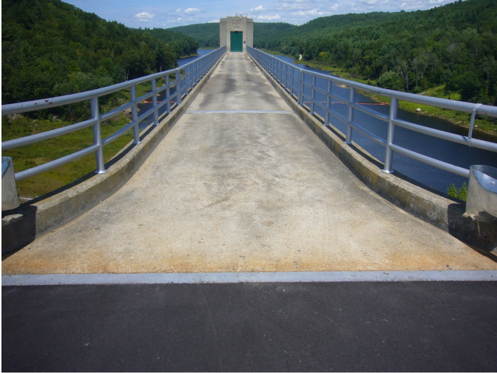
Photo 9: Otter Brook Lake Service Bridge – Plan View
