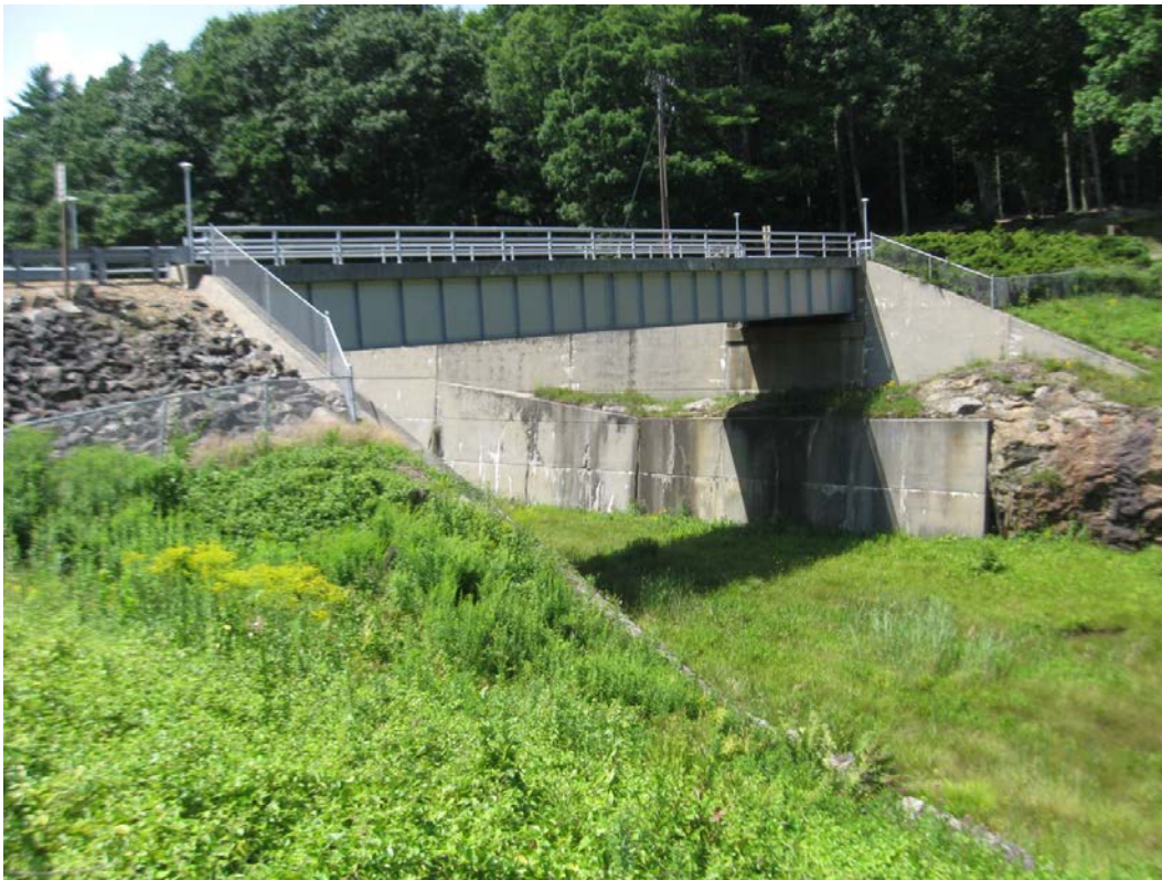
Photo 14: Barre Falls Dam Spillway Bridge – Elevation View
