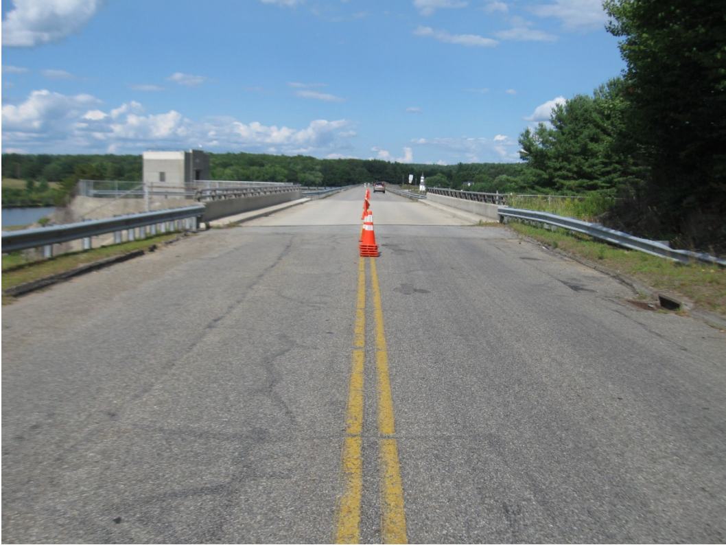
Photo 21: W. Thompson Lake Spillway Bridge – Plan View
