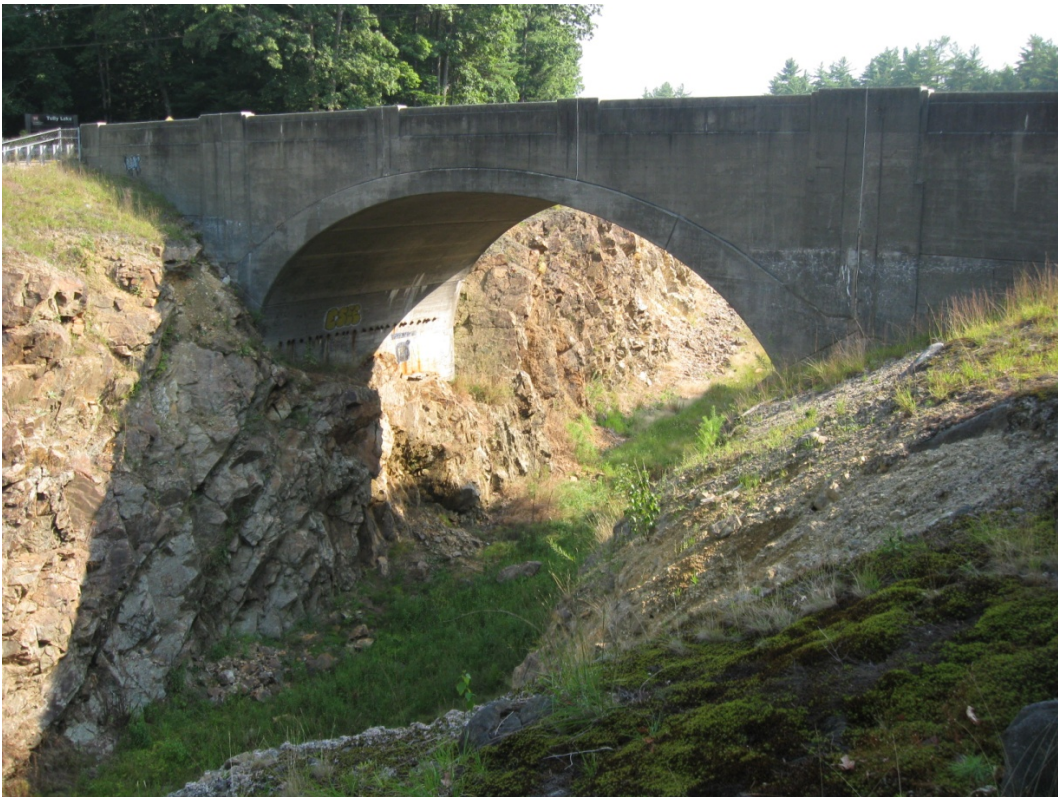
Photo 12: Tully Lake Spillway Bridge – Elevation View
