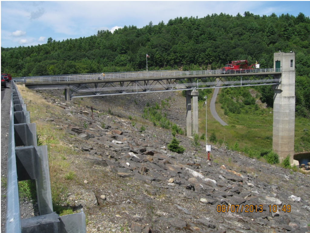
Photo 10: Otter Brook Lake Service Bridge – Elevation View
