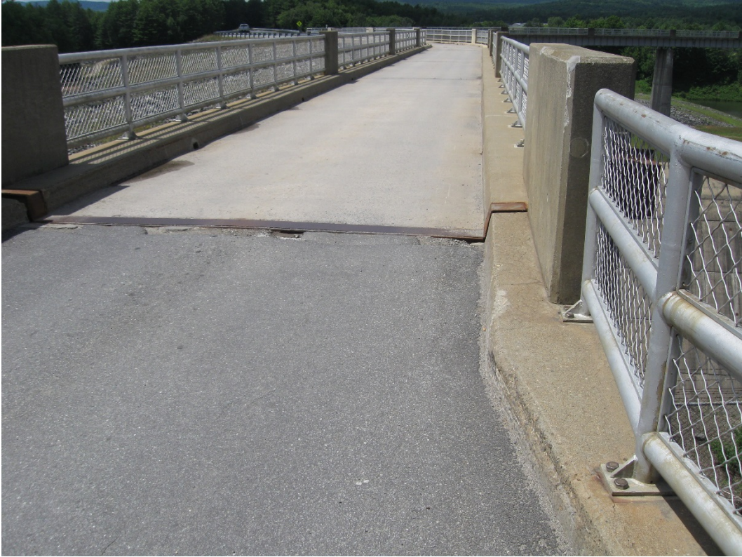
Photo 1: N. Springfield Dam Spillway Bridge – Plan View
