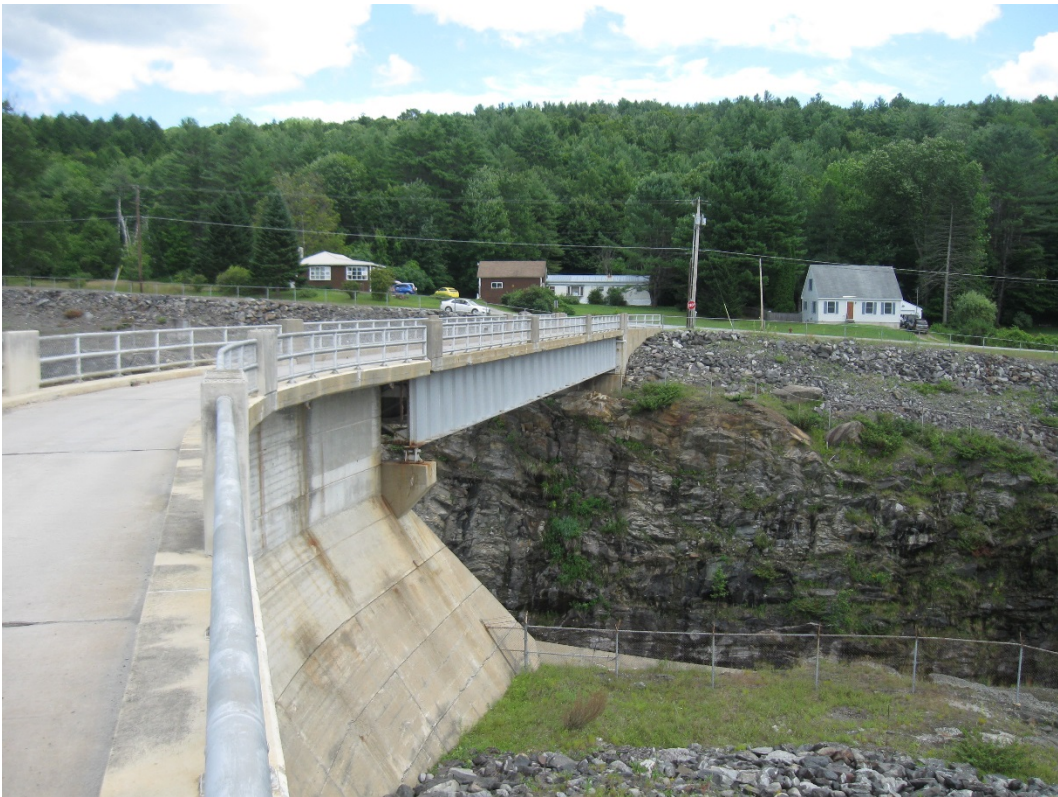
Photo 2: N. Springfield Dam Spillway Bridge – Elevation View
