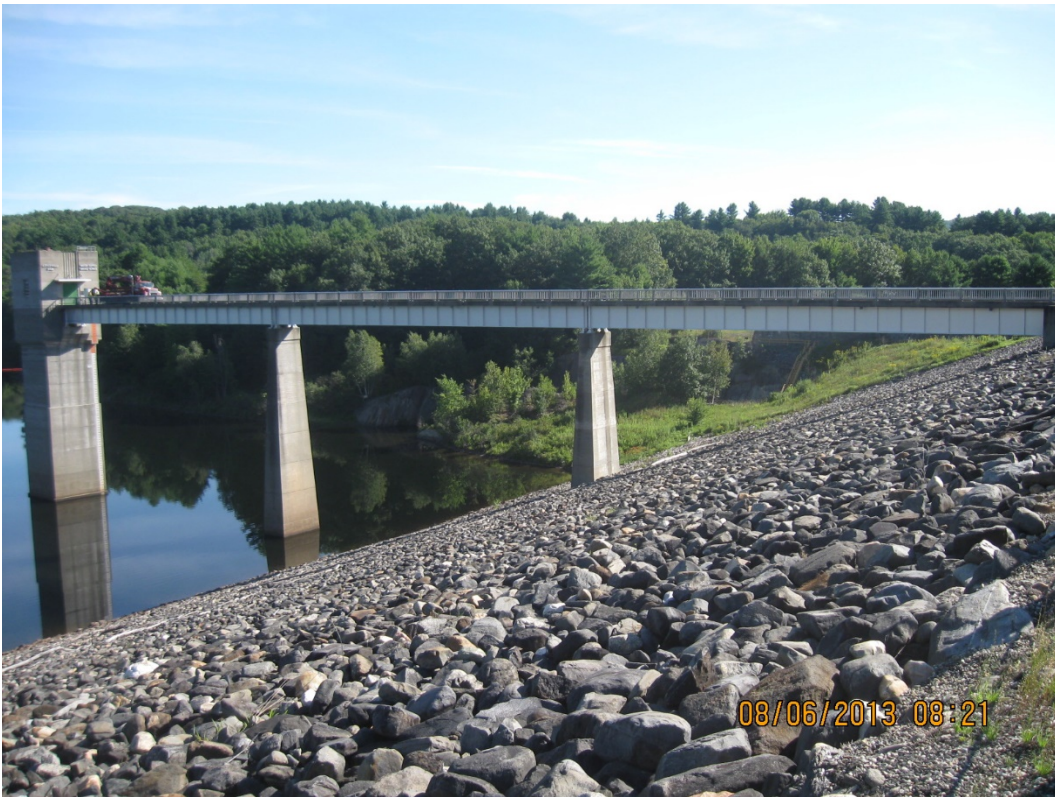
Photo 18: Littleville Lake Service Bridge – Elevation View
