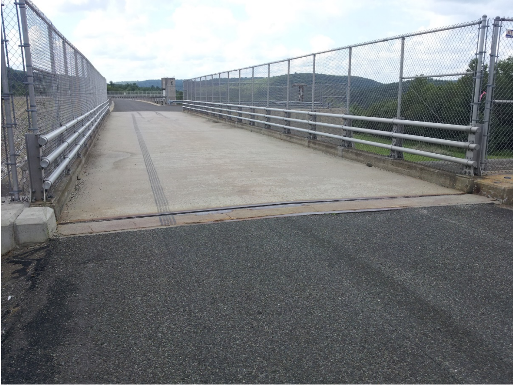
Photo 23: Thomaston Dam Spillway Bridge – Plan View
