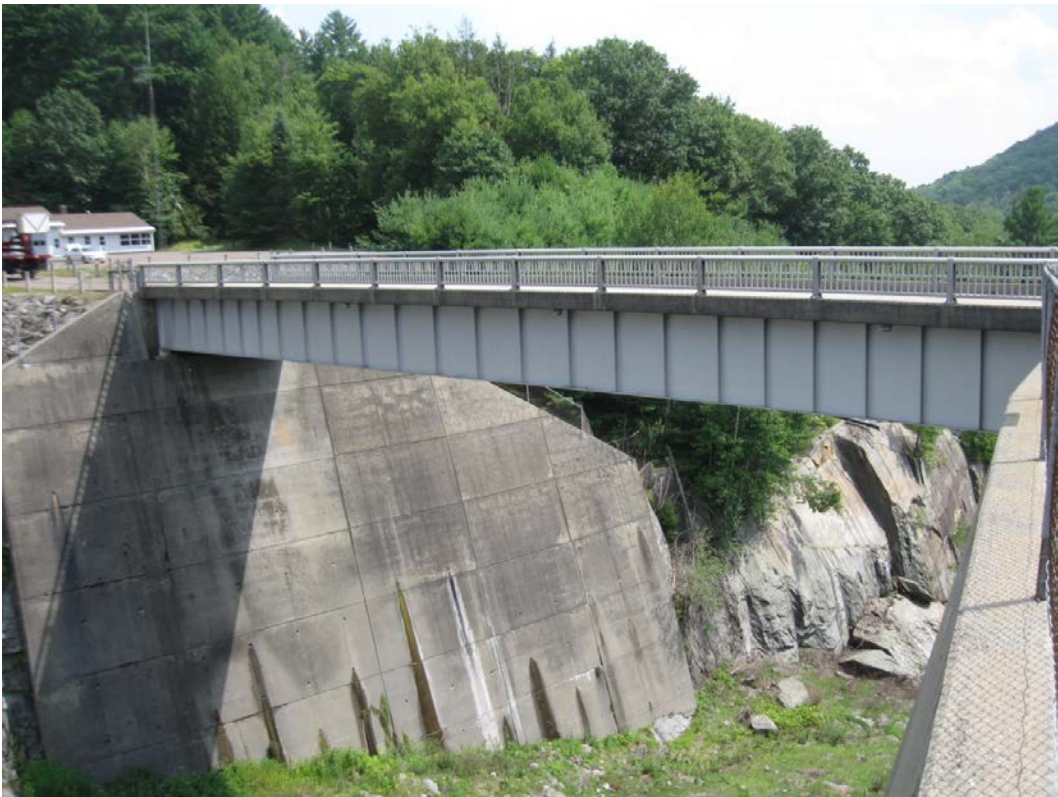
Photo 20: Littleville Lake Spillway Bridge – Elevation View
