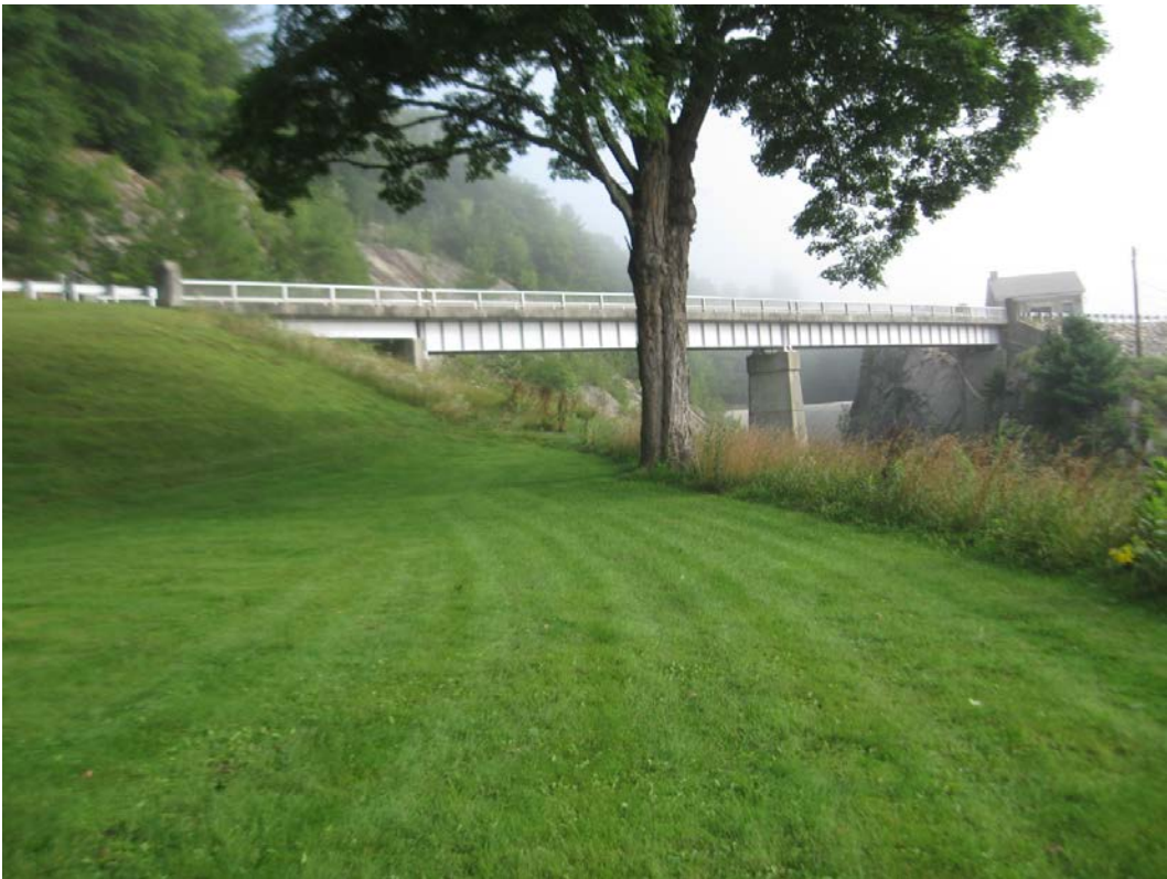
Photo 6: Surry Mountain Lake Spillway Bridge – Elevation View
