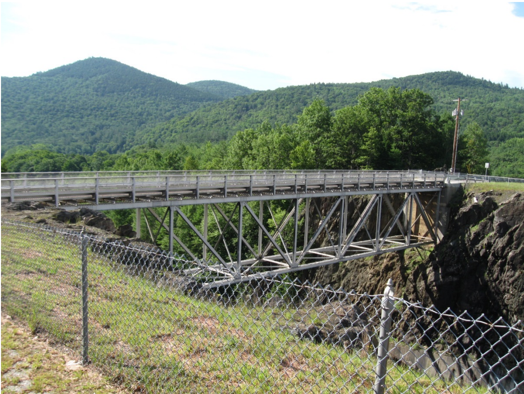
Photo 4: Townshend Lake Spillway Bridge – Elevation View
