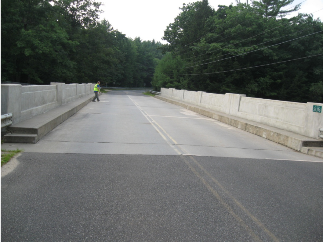
Photo 11: Tully Lake Spillway Bridge – Plan View
