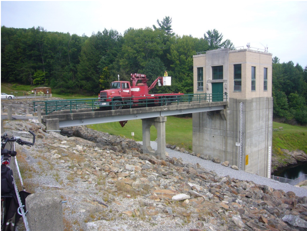
Photo 8: Edward MacDowell Lake Service Bridge – Elevation View
