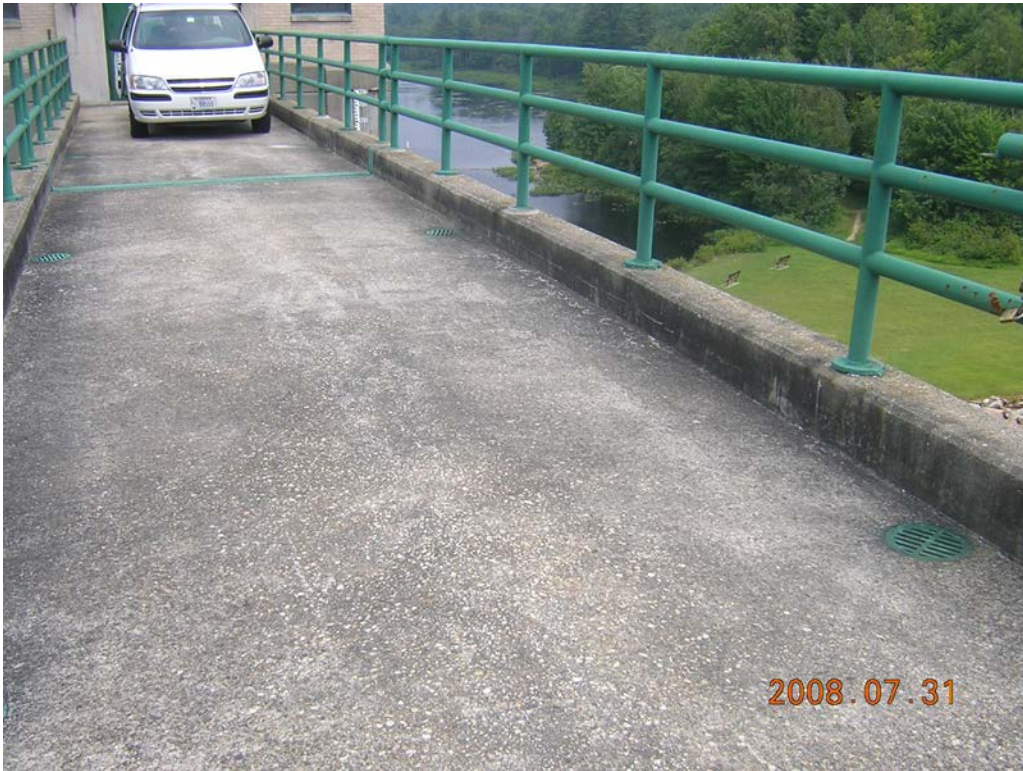
Photo 7: Edward MacDowell Lake Service Bridge – Plan View
