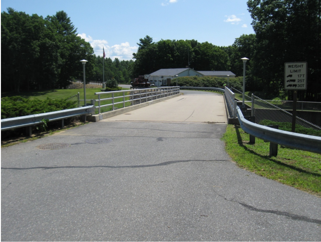
Photo 13: Barre Falls Dam Spillway Bridge – Plan View
