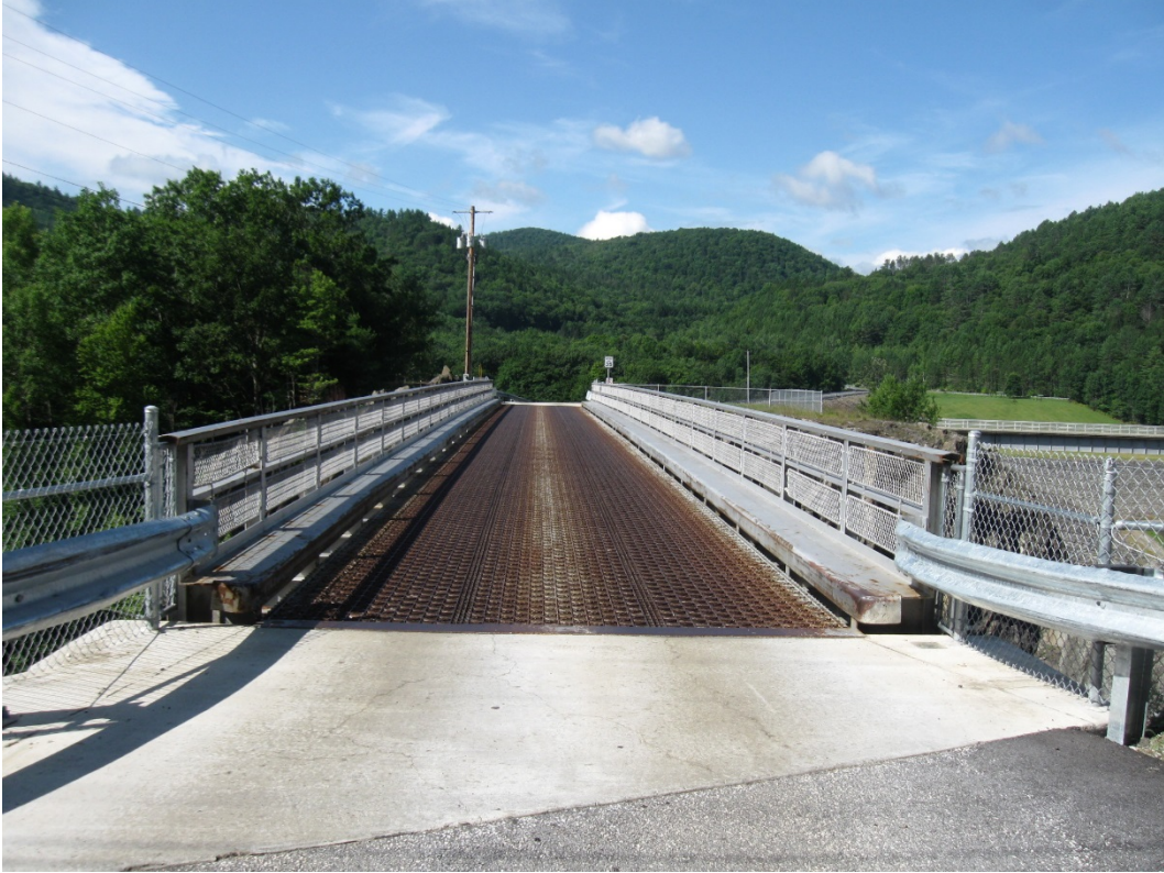
Photo 3: Townshend Lake Spillway Bridge – Plan View
