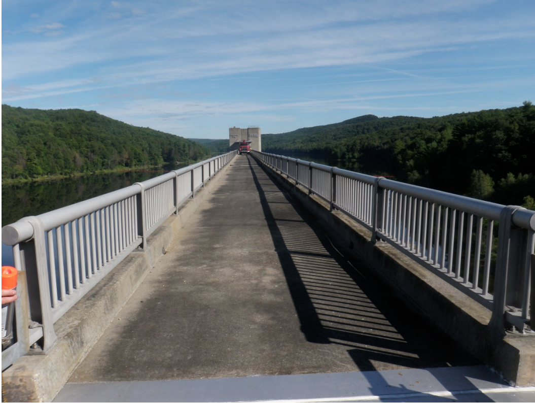
Photo 17: Littleville Lake Service Bridge – Plan View
