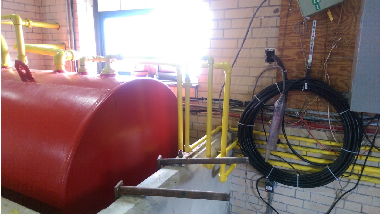
Informational Photo Number 2: Fuel pipe connections
