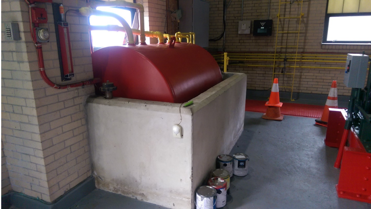
Informational Photo Number 1: Overview of tank.
